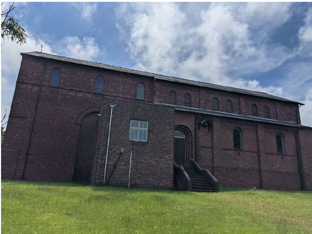
Fig. 3 | Church Photographs (3.1 + 3.2 Exterior)
