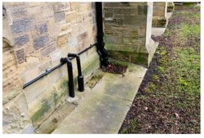
Gas incoming supply and pipe to the basement boiler room.
