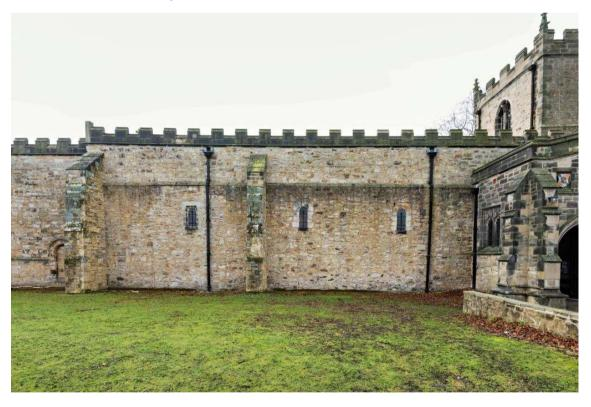
North Elevation of Nave: oldest masonry below the string line.
