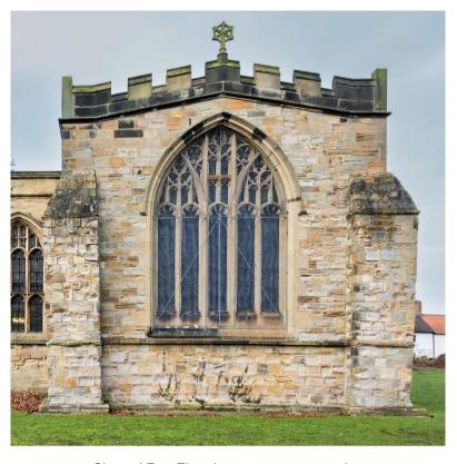
Chancel East Elevation: severe stone erosion.
