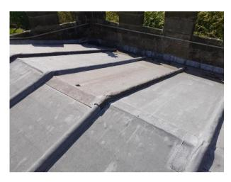
Tower Roof: Lapped ridge with patch repairs
