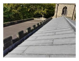
Nave roof south pitch in lead rolls with ventilated ridge and south aisle in stepped bitumen felt
