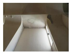
Photo 31, Example of lifting paint and staining to ceiling
