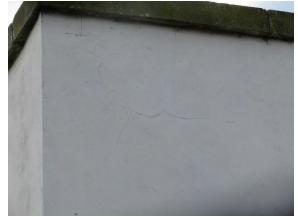
Photo 12, Crazed cracking to render
