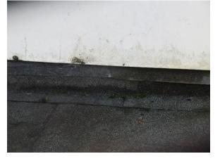
Photo 14, Example of vertical cracking over drip bead over flat roof
