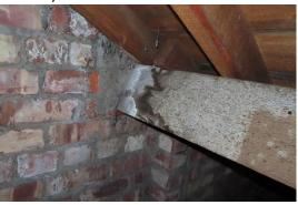
Photo 28, Evidence of water staining to purlin ends
