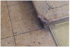
Photo 38, Damage to corners of altar platform
