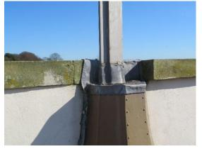
Photo 21, Lead capping to cross base
