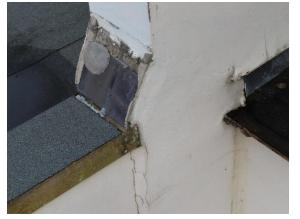
Photo 19, Cracked render and slipped slates at junction to vestry parapet
