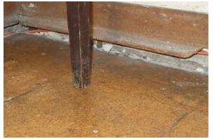
Photo 37, Gap between skirting and floor in SE corner
