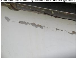
2.4.8 Horizontal cracking below rainwater gutters.
