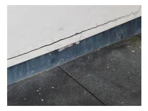
Photo 16, Example of horizontal cracking over lead flashing over flat roofs
