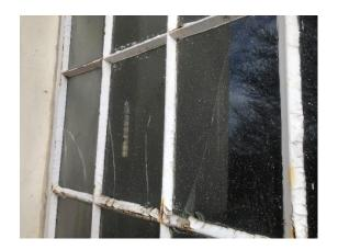
Photo 26, Example of broken window glazing
