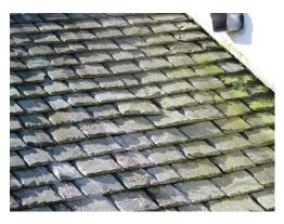
Photo 2, Example of slipped slate to north elevation
