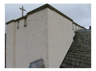
Photo 13, Cracking to south face of tower
