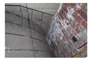
Photo 35 Salt deposits on inside brick face. Metal frame and mesh structure of barrel ceiling
