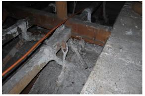
Photo 29, Broken support for fibrous plaster of vaulted ceiling
