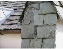
Photo 4, Example of slipped slate to buttress
