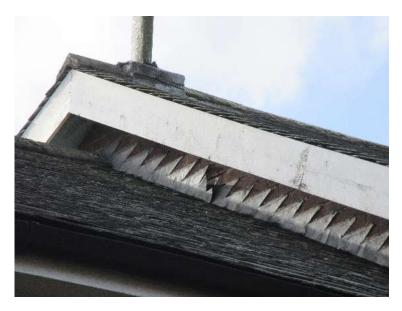
13. Small flat roofs at NW (open Porch) and SW (we off Narthex) abut the brick walls. Copper with capped battens, covered with non-setting deterrent and disguise paint. Pitched capping on Tower similar copper but unpainted. All appear sound.
