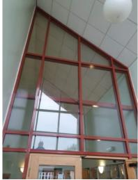
b) A suspended ceiling follows the slope of the roof structure.
