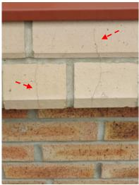
b) Micro-fractures in the cant bricks forming cills
