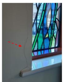
b) Cracked plaster to the left-hand side of the cill
