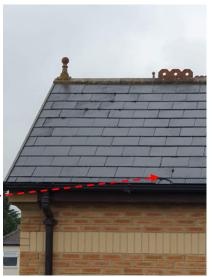
b) Cracked slate directly above the guttering
