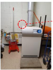
a) Boiler. Note the long vertical crack in the wall behind and to the left of the boiler
