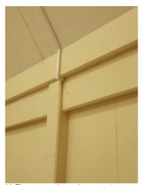
b) The post and panel structural system of the 1950s church is a visible part of the interior.
