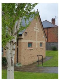
b) Brick 'specials' to for crucifix in the east elevation of the nave/ vestry.
