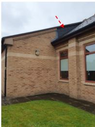
a) Abutment flashing where roofs of differing pitch intersect
