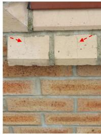
a) Micro-fractures in the cant bricks forming cills
