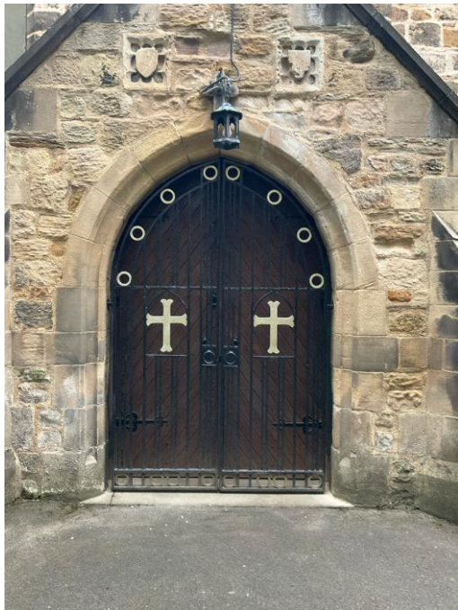
Porch Door with metal security gates
