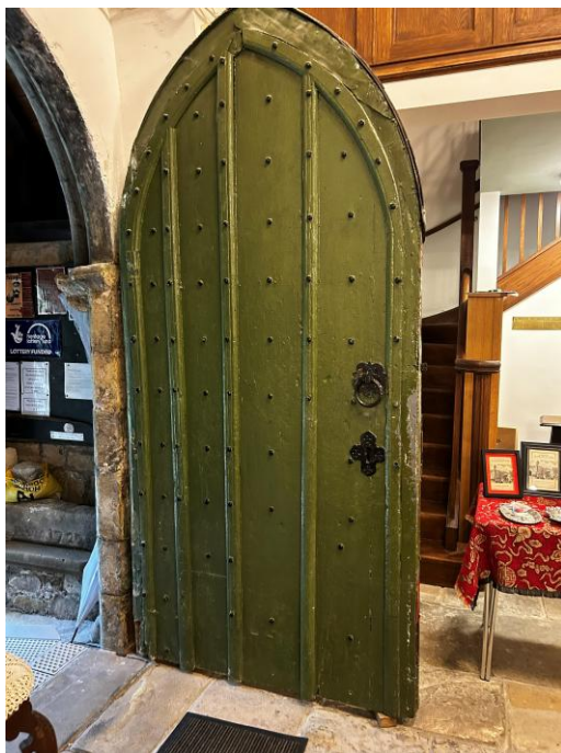
Internal Porch Door
