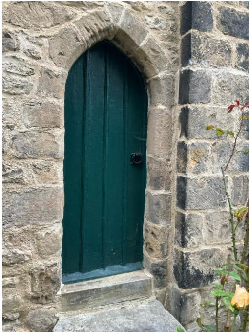
Chancel south door
