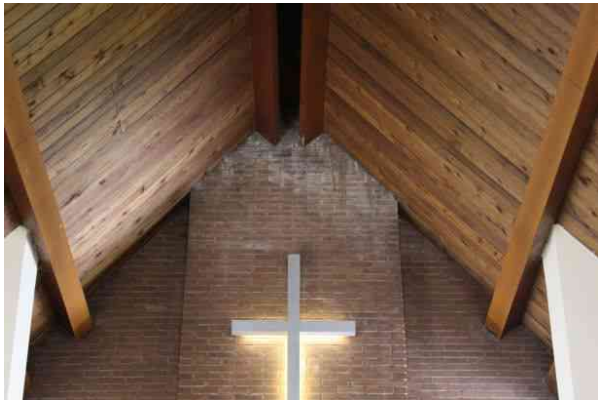
Staining from water leaks at roof/ gable stack
