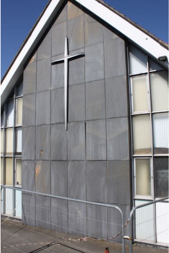
Loose slate cladding to south gable
