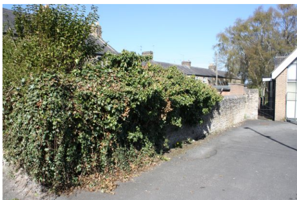
Shrubs in need of pruning
