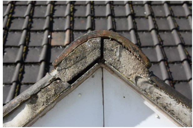
Cracked mortar bedding to gable ridge
