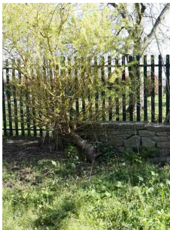
Shrub causing cracking of dwarf wall
