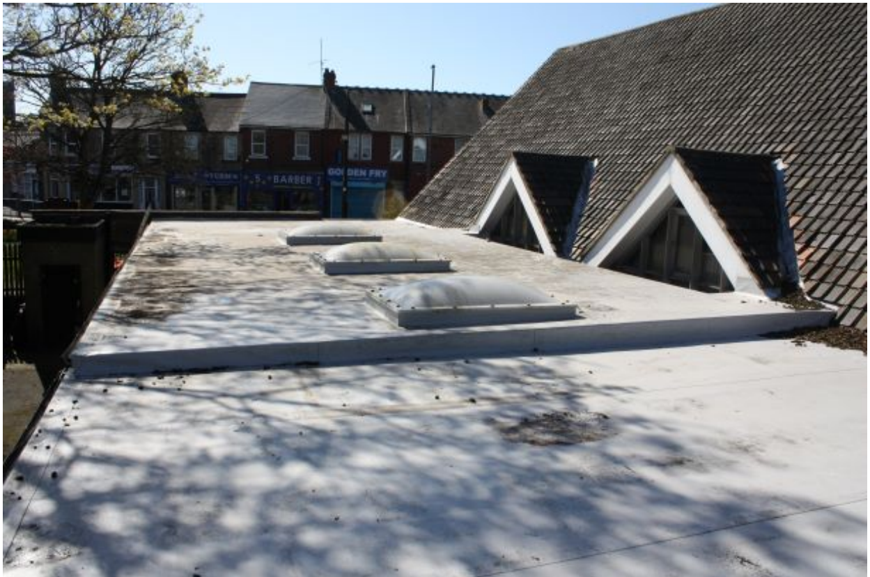
Flat roof of Hall block and pitched roof of Nave showing volume of water discharging into narrow gutters
