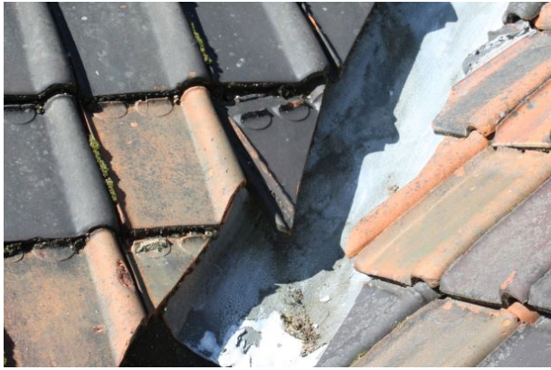
Loose valley tile
