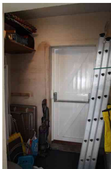
Escape door needs adjustment
