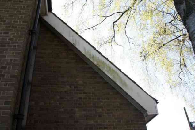
Green staining of gable fascia
