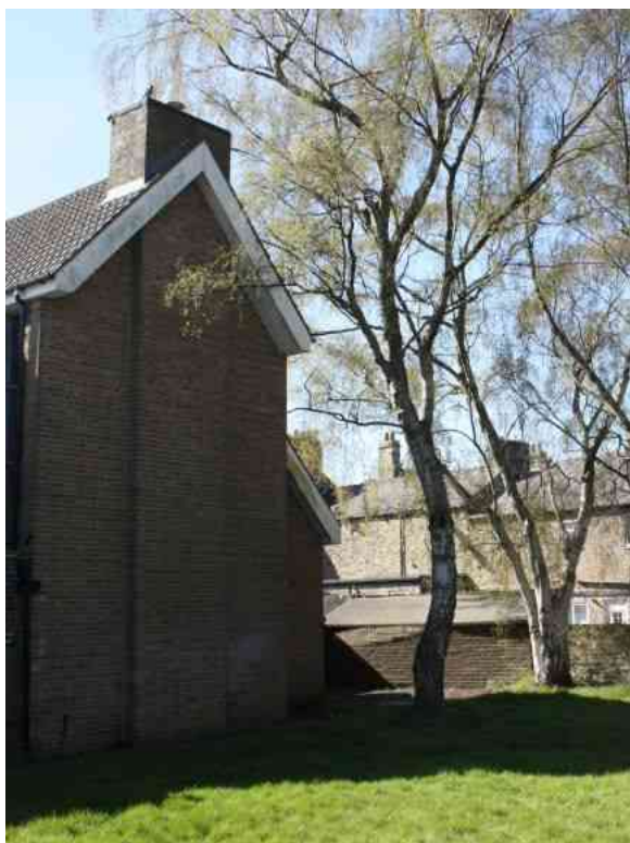
Mature silver birch tree near north gable resulting in stepped cracks to NW wall
