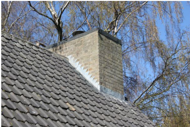
Chimney stack with torn flashing to coping
