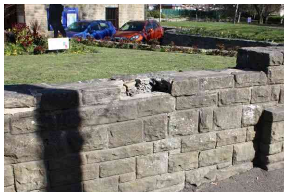
Missing coping to dwarf wall adjacent road
