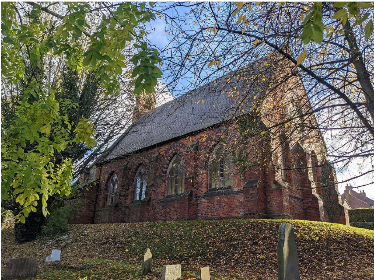
Fig. 4 | Church Photographs (4.1 + 4.2 Exterior)
