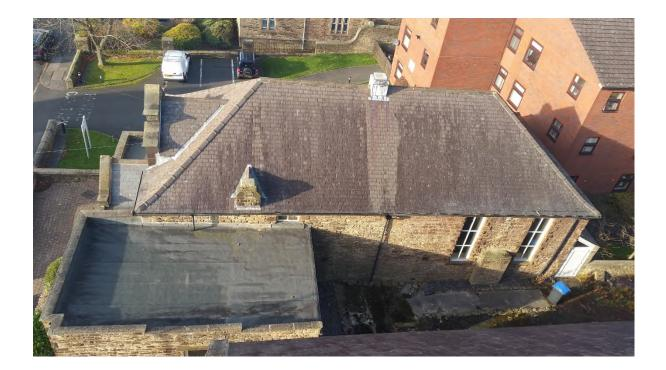
Walls have got cement ribbon pointing and there is an area of walling that is poor. Walling is coursed but generally ok on the road side elevations, there has been some cement repairs that is not very good.
