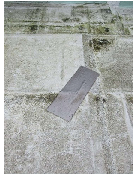
Flashband patch on Sarnafil
