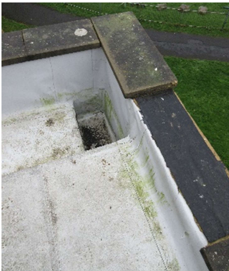
Felt patch where copings missing
