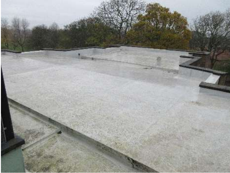
Sarnafil roof carried over designed gaps in coping
