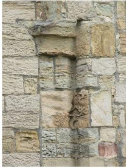
Blocked arch at E end of N Aisle by the Lambton stair – decayed but no visible change
