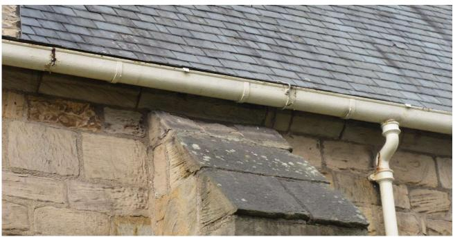
S Aisle W end – gutter and pipe breaks
