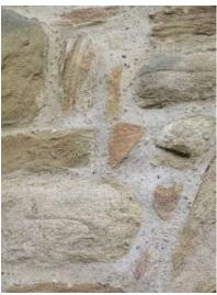
Mixed stone and pointing types W side of Tower – including recent lime pointing over the W door
