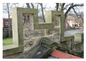
42. S Aisle W gable including its N buttress – many stones including the buttress have slight surface decay behind hard dark pointing. Scattered pocket decay especially close to the top of the gable.
