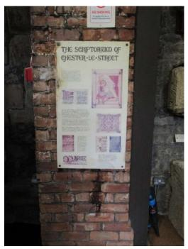
Brick Chimney where it passes through the Ankerage salts continue to effloresce full height especially at top and now tarry water seeps out at head height
