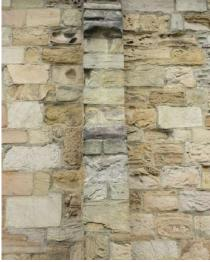
S Aisle – decay at buttress E of the Porch
