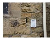
38. Nave E gable – fair but deep decay at isolated stones near the peak and holes in the pointing especially low on the S side.
