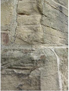
Corner S of the W face – joints cracked above and below rusting channel end
