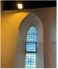
Figure 24 – window with hopper and cracked pane
