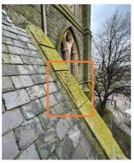
Figure 4- Coping stone delamination
