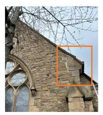
Figure 8 - crack to kneeler at 8.4.1
