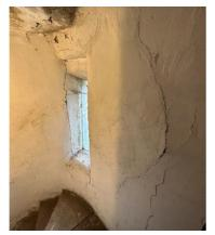
Figure 15 - crack to stair
