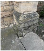
Figure 9 - erosion to base of buttress
