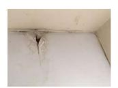
Lath and plaster ceiling above Narthex north lobby is water damaged. Repair after roof is recovered (9.1.2).
