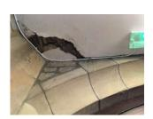
4. Vaulted lath & plaster above Narthex is suffering from water ingress.
