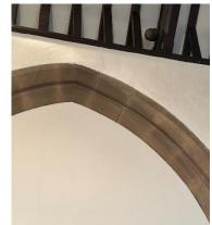
Figure 26 – Arcade open joint
