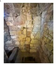
Figure 13 – Crack to E side belfry
