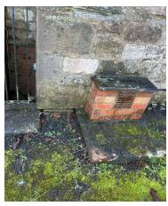
Figure 18 – Former Coal Chute
