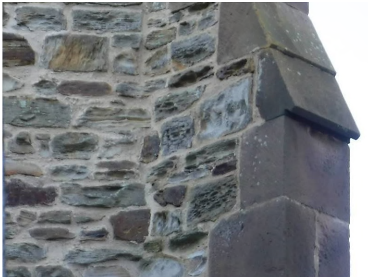
Some slight honeycombing to the stonework on the North East buttress.
