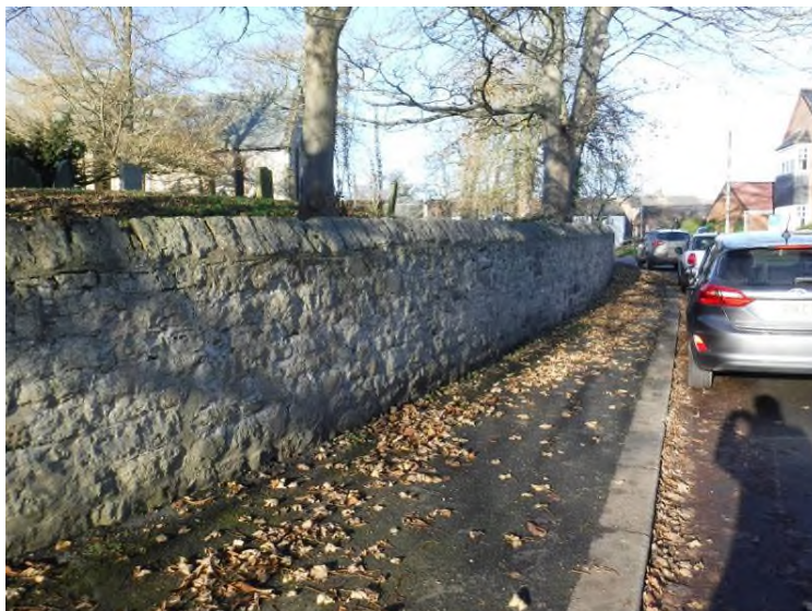
Wall bulging out a bit on the East end where there is a cut down bit of a tree which they haven't completely killed off.
