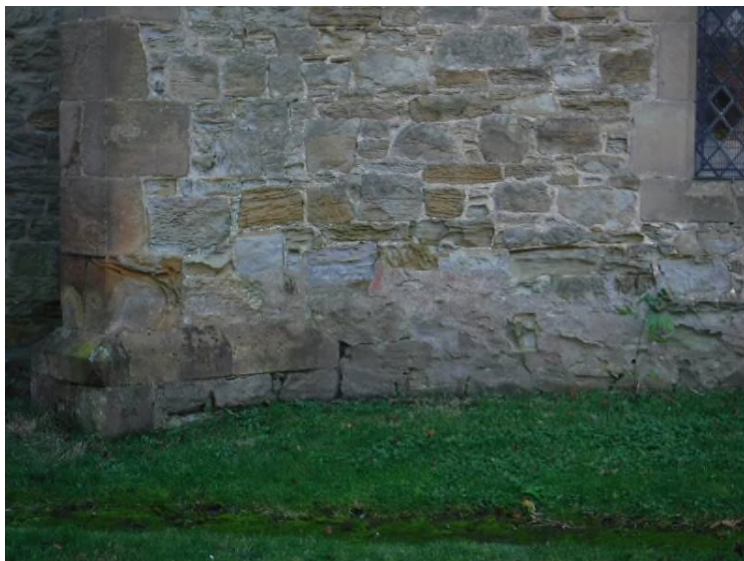
Some slight open joints by the North East buttress both buttresses, there is also the start of a plant growing that needs to be removed, and also there is an area of rendering which is probably hiding poor quality stonework.
