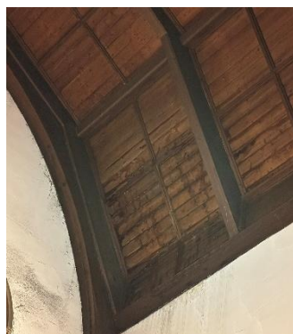
Figure 37 – Chancel South roof
