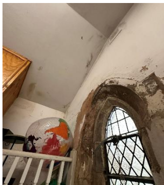
Figure 62 – Vestry ceiling and E
