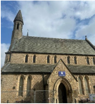
Figure 4- South Nave and Aisle
