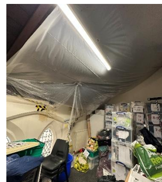
Figure 58 – ceiling S aisle W end
