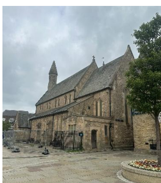
Figure 38 – new fence and gravel
