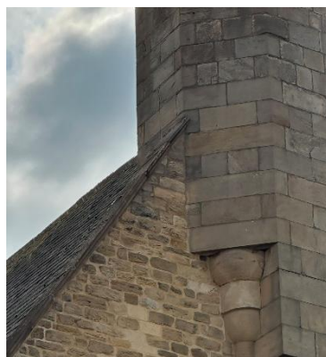
Figure 2 – Coping to NW Nave
