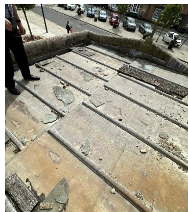
Figure 8 – SE lead roof (over WCs)
