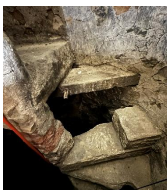
Figure 67 – missing step
