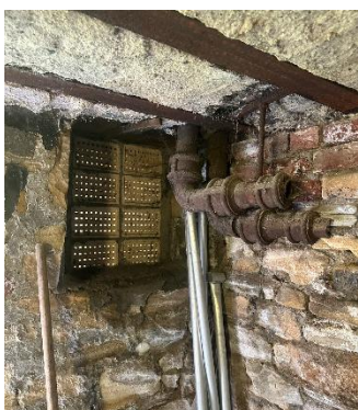
Figure 31 – ceiling and former window
