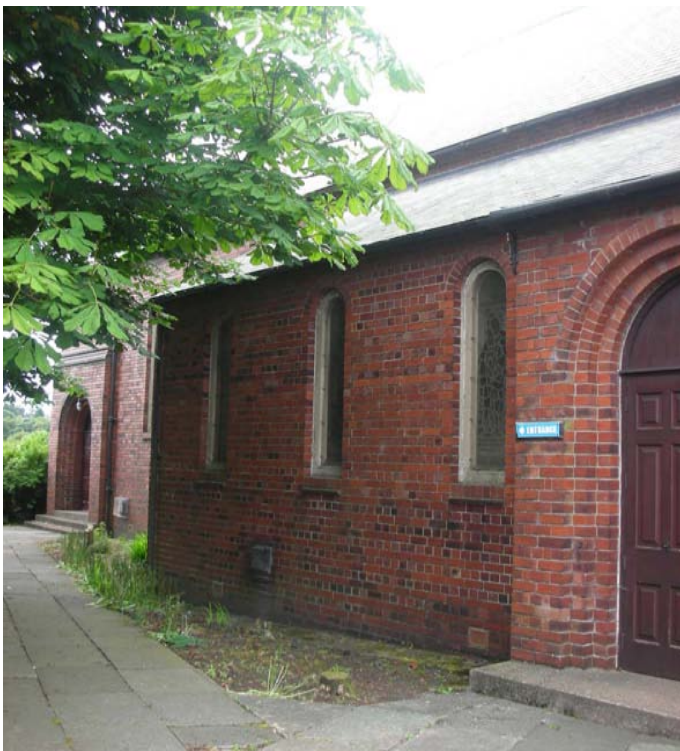
Pathways in reasonable condition, vegetation close to external wall
