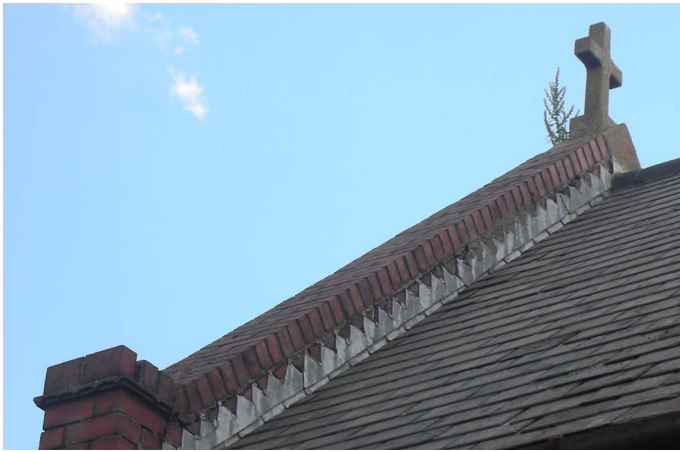
Upstand parapet of chancel gable has open joints, allowing water ingress. Cement smeared over flashings on west pitch (below) will be holding water
