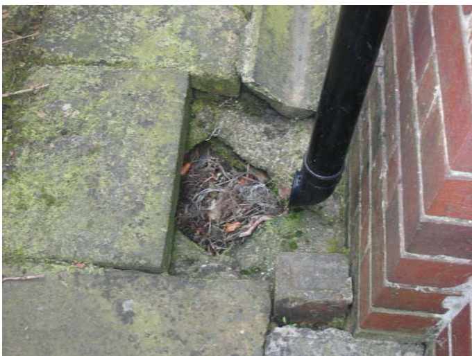
Blocked gully with no guard
