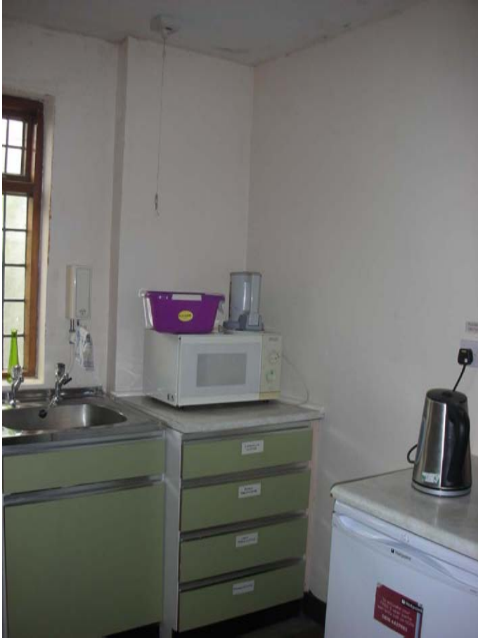
Signs of (historic?) water penetration over windows, and current evidence of black condensation mould above kettle
