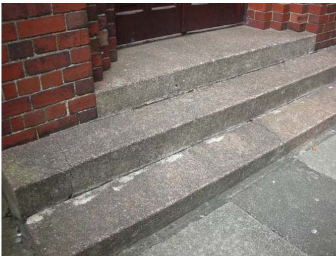
Substantial cracks in steps to south east porch
