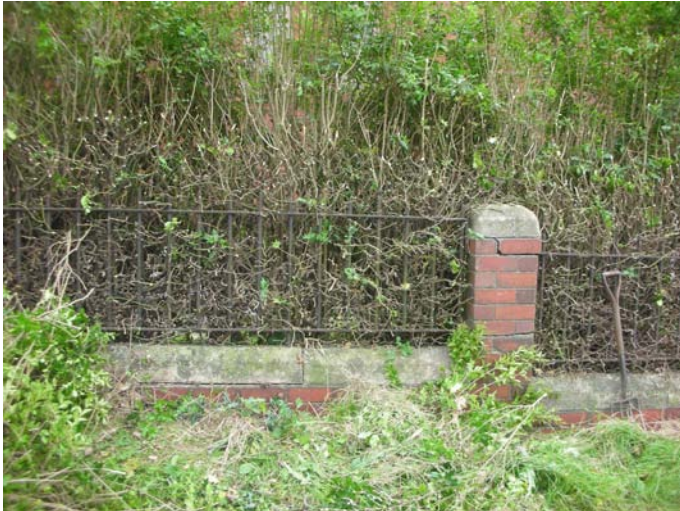
Boundary walls dislodged by vegetation
