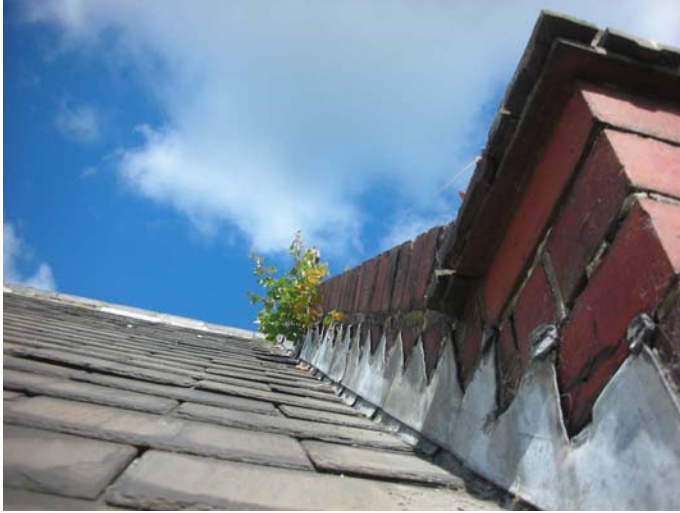
Upstand parapet of chancel gable has open joints, allowing water ingress. Cement smeared over flashings on west pitch (below) will be holding water
