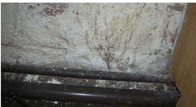
Possible signs of wet rot, damp timbers & wet ground
