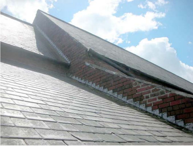
Slating in reasonable condition, re-pointing to nave and aisles and to verges in cementitious mortar
