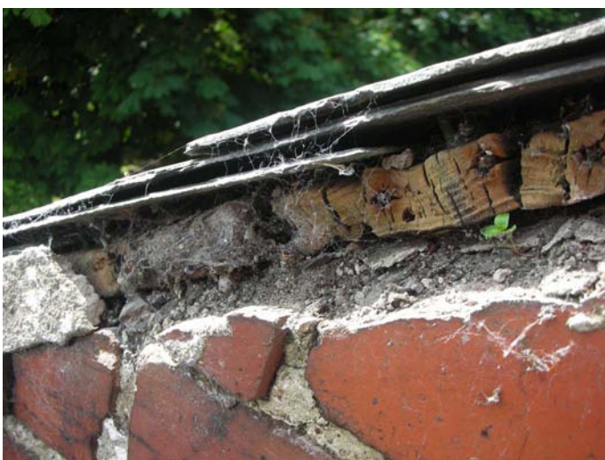
Cementitious mortar fillet to verge cracked, failed and detached
