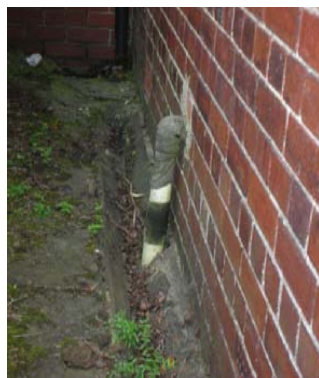
Flags and drainage channels against external wall will be holding water in the base of the wall
