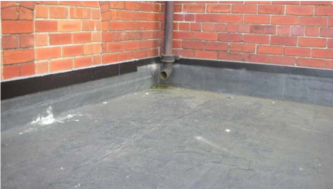
Kitchen re-roofed recently in single-ply membrane - good condition
