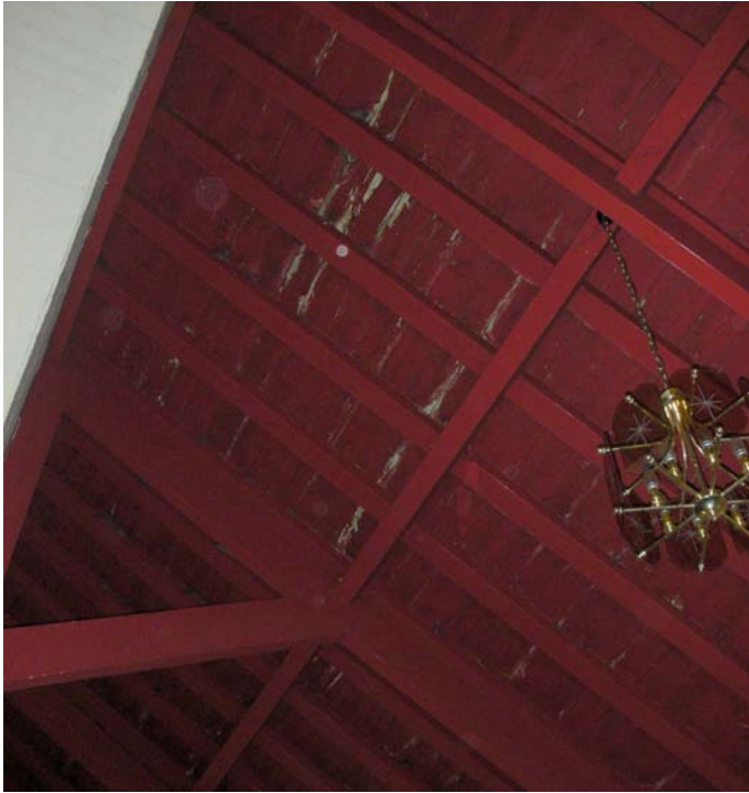
Exposed roof structure to aisles - evidence of water ingress
