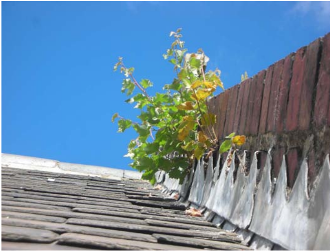
Open joints to flashings supporting vegetation
