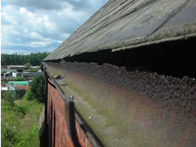
Cast iron gutters rusting
