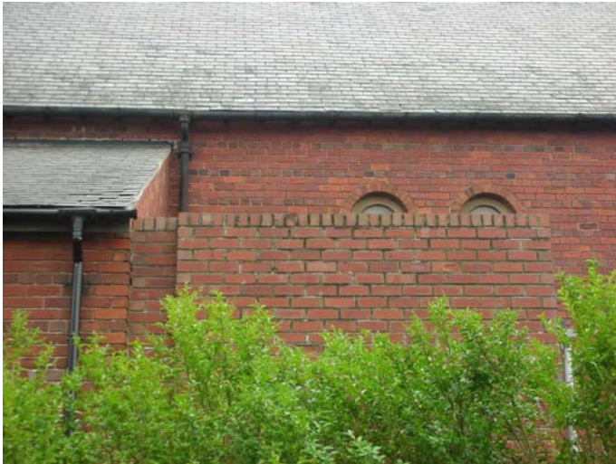
Kitchen extension - open joint to abutment with west aisle (meeting room), and signs of damp brickwork at high level
