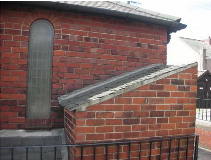
Flashband to steps and boiler house roof to be monitored
