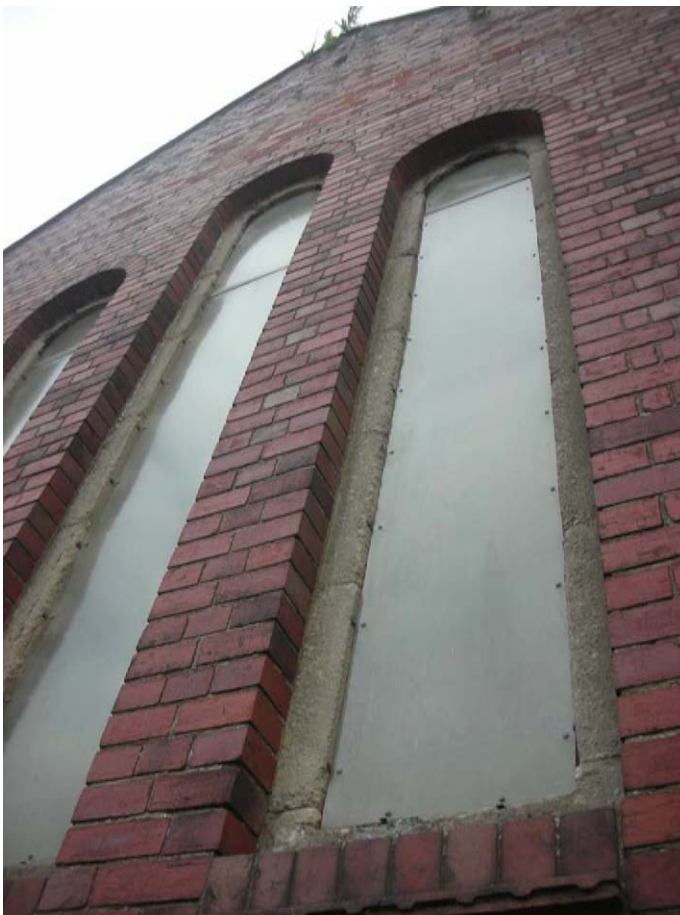
Replica reconstituted stone reveals deteriorating, ferrous fixings for polycarbonate sheets are rusting and polycarbonate is now cloudy and yellowing with age
