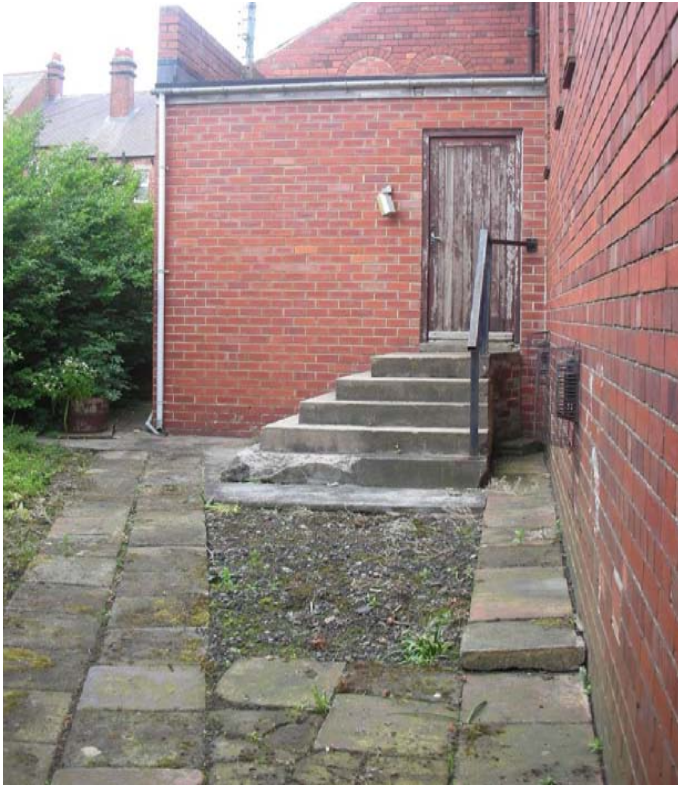
Pathways to west uneven but serviceable, kitchen steps in poor condition
