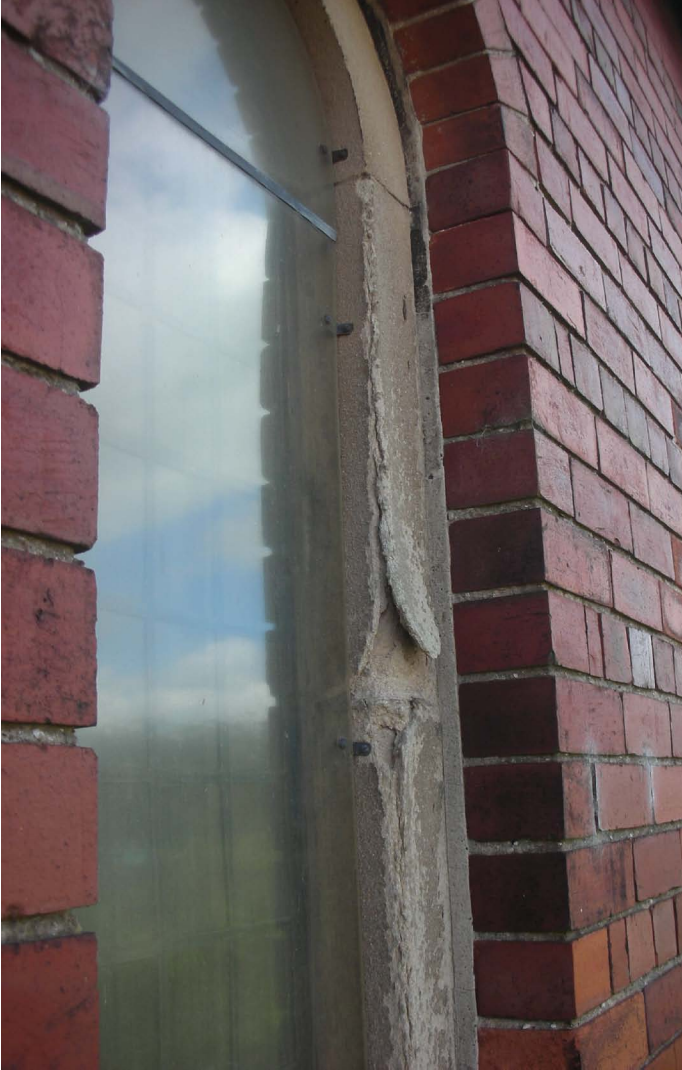
Spalling of reconstituted stone reveals
