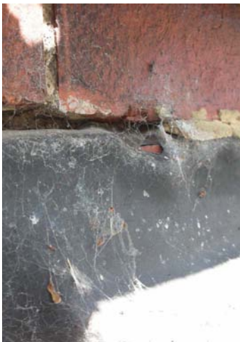
Loose, ripped and split flashings
