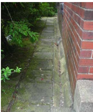
Flags and drainage channels against external wall will be holding water in the base of the wall
