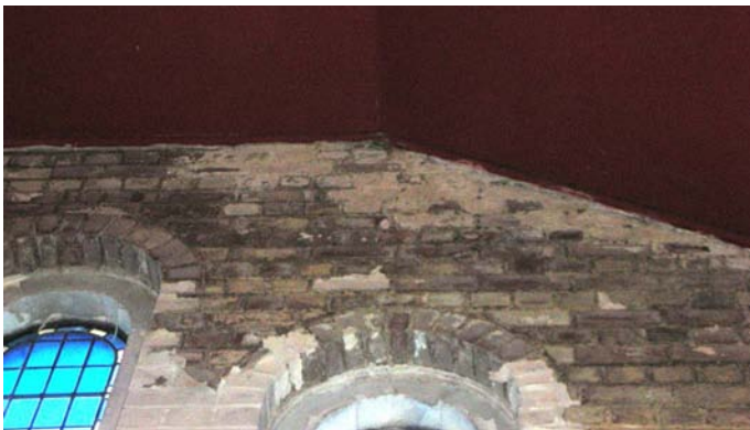
Friable paintwork and salt damage to brickwork, above and below.
