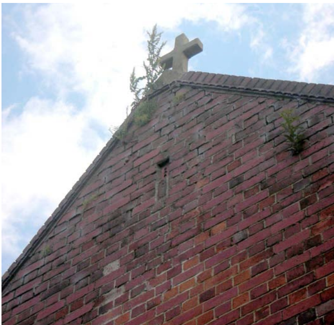
Deteriorated pointing and damaged brickwork to chancel gable
