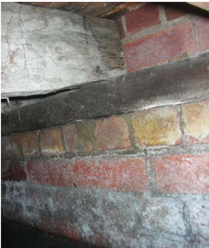
Possible signs of wet rot, damp timbers & wet ground
