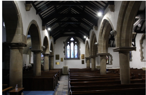
View of Inner Aisle to west
