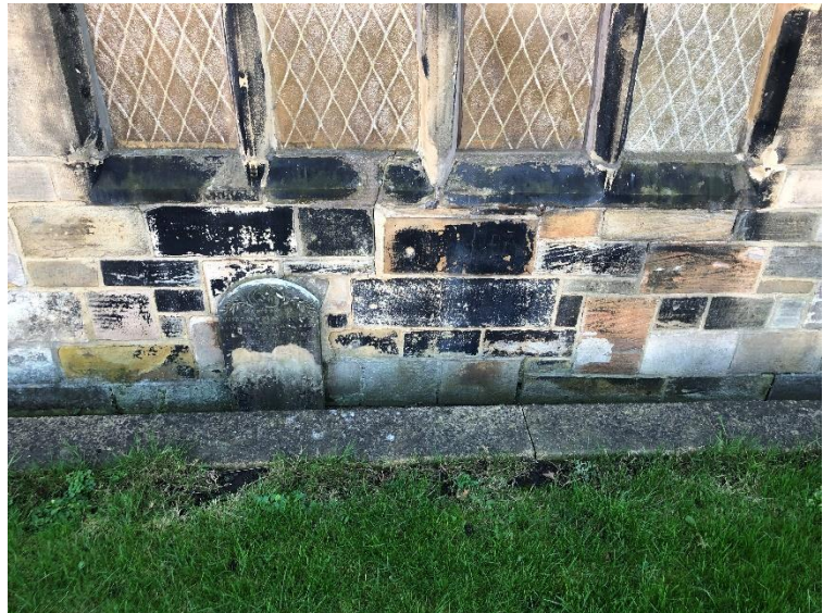
Fig 5. Window detail showing glazing and repointing to Choir Vestry
