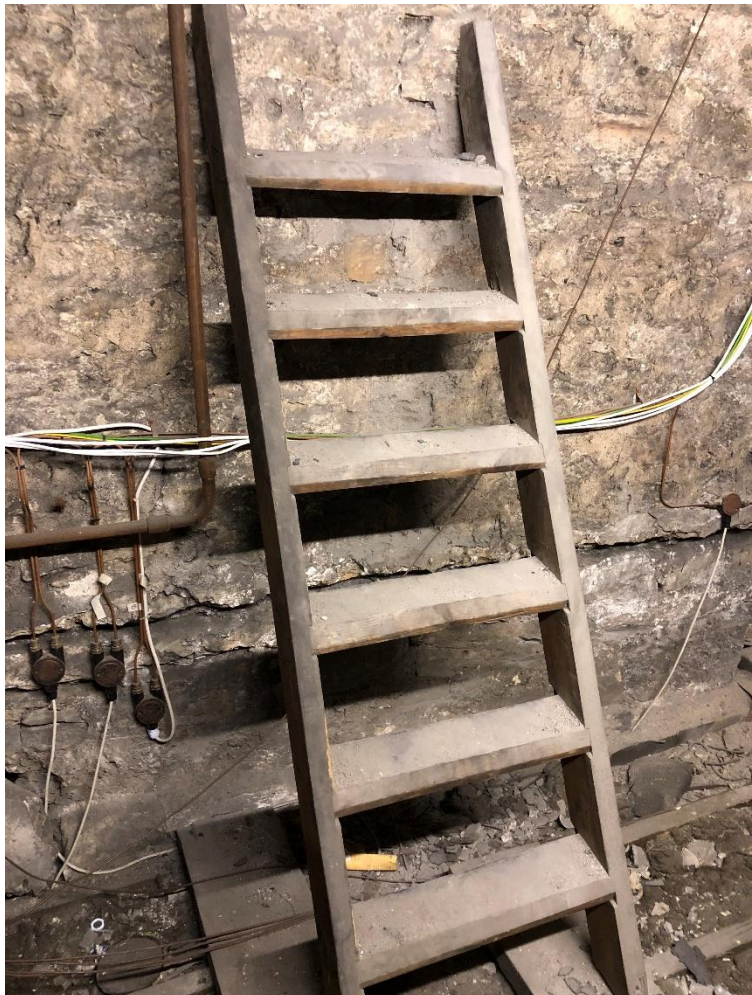
Fig 15. Access ladder, north aisle roof void
