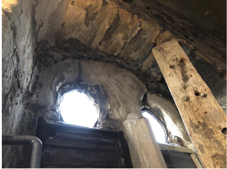
Fig 11. Western Belfry opening prior to mullion removal
