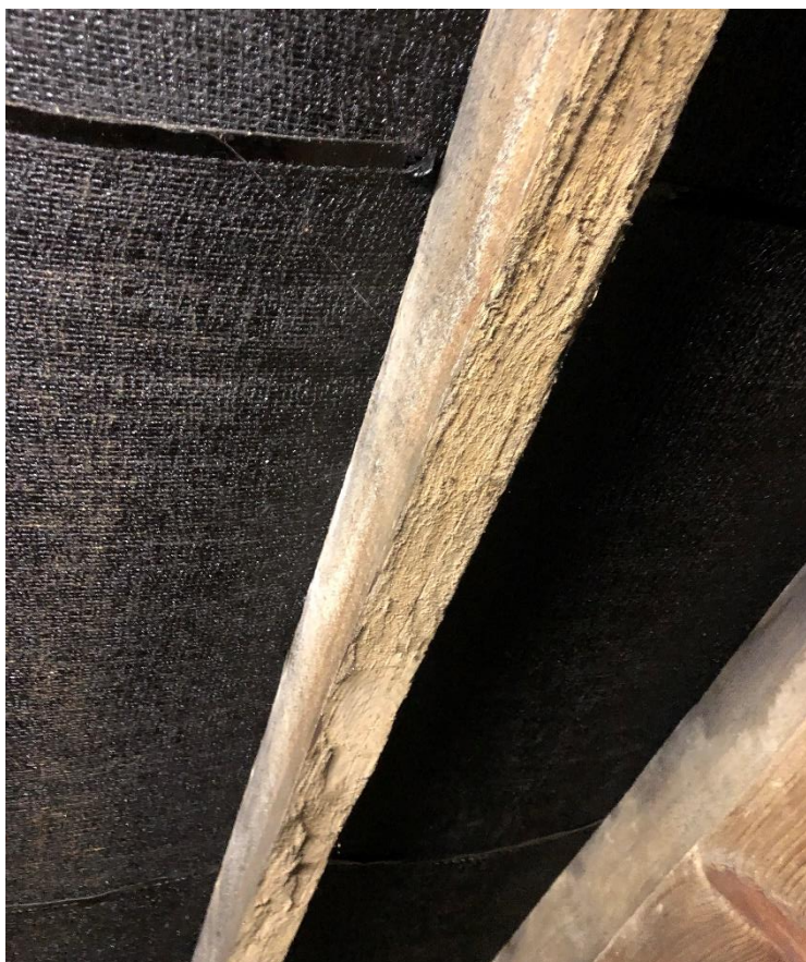
Fig 19. Loft space, exposed timber
