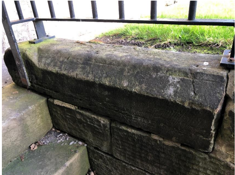
Fig 20. Steps to boiler room; stonework to wall
