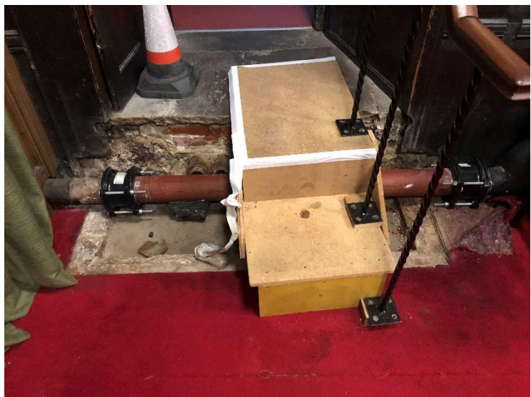
Fig 13. Replacement steps/handrail to kitchen (pipework repair)
