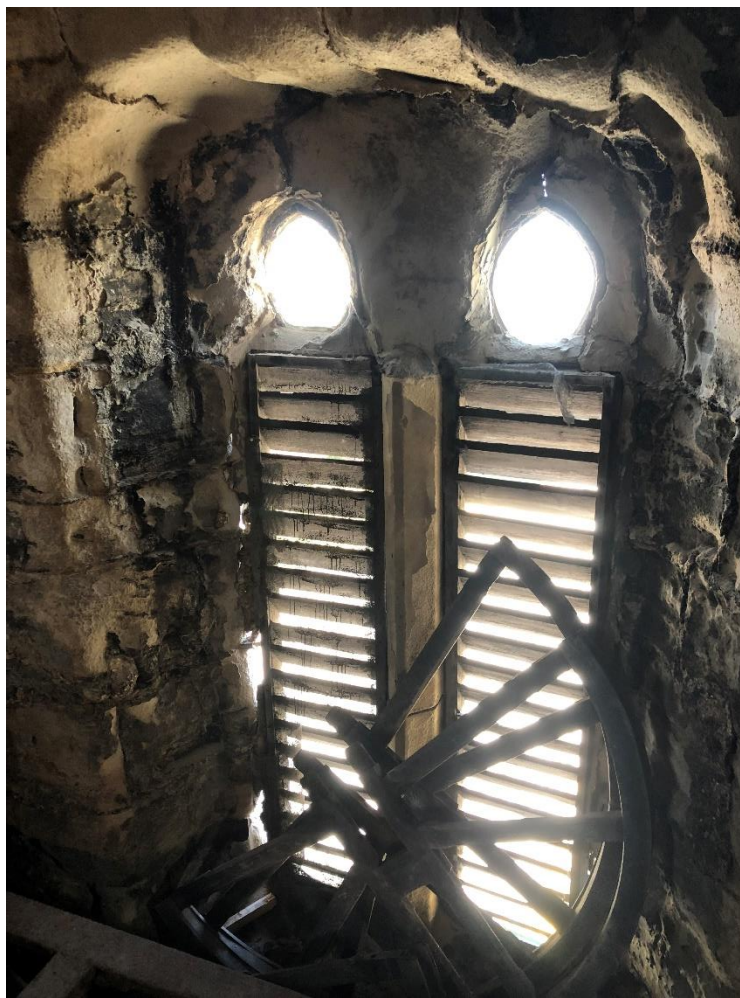
Fig 18. Belfry openings with louvres (internal)
