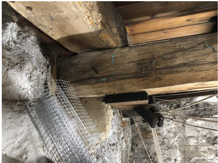
Fig 12. Check woodworm treatment (Tower)
