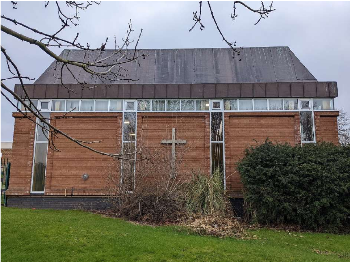
Fig. 3 | Church Photographs (3.1 – 3.4 Exterior)
