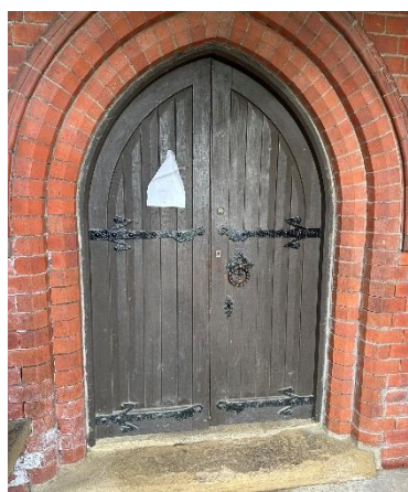
Figure 13- Main entrance doors
