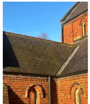
Figure 3- Porch east roof
