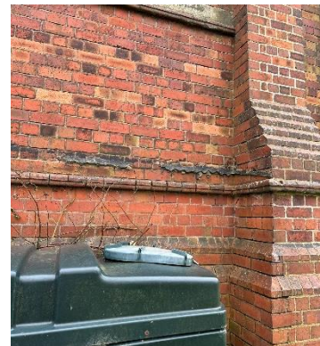
Figure 10 – Former lean-to flashing
