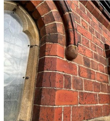
Figure 6 – Window Reveal S Aisle
