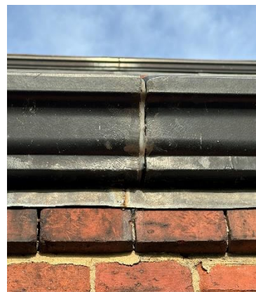
Figure 4 – Gutter joint to S Aisle
