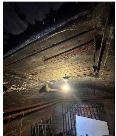
Figure 15 - Hatch to boiler ceiling
