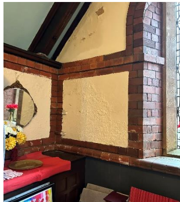
Figure 24- SW end of S Aisle
