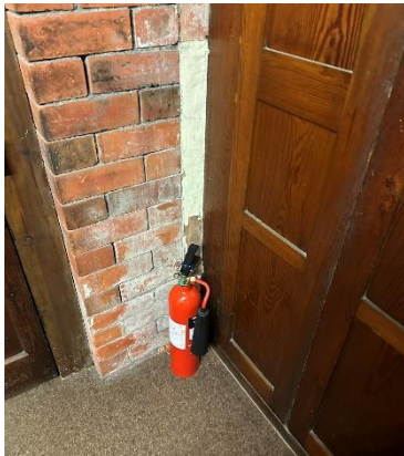
Figure 26- Efflorescence near office lobby
