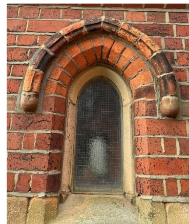
Figure 12 – East Porch window
