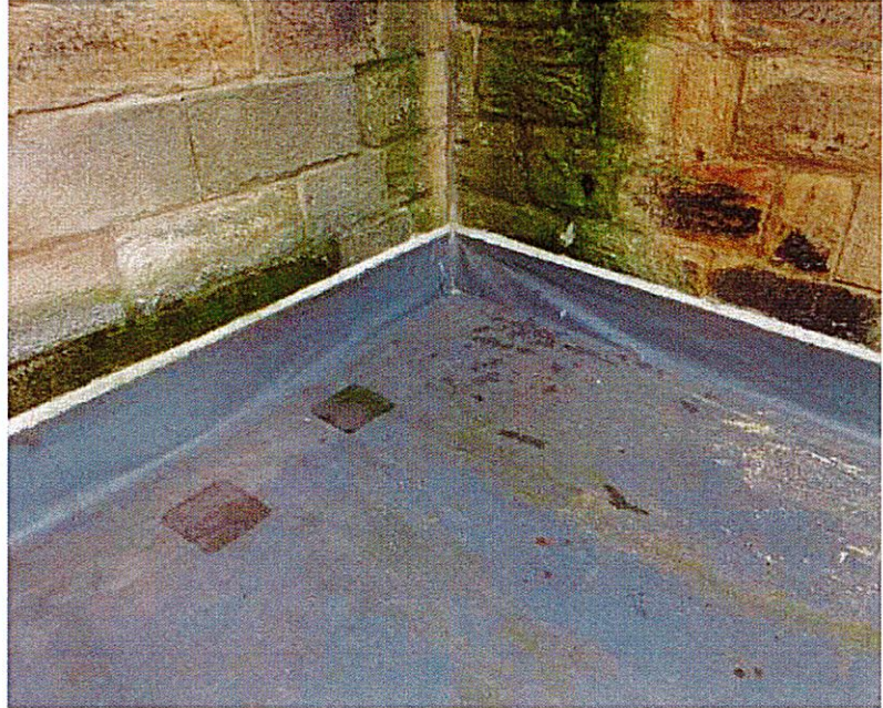
Wet wall over Vestry
