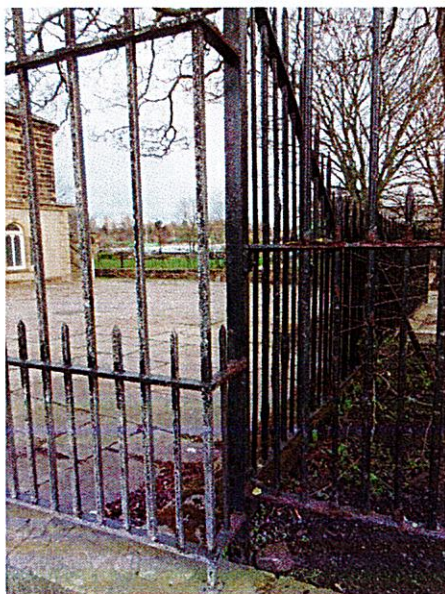
Painted galvanised N railings at L, earlier unpainted now delaminating churchyard railings at R
