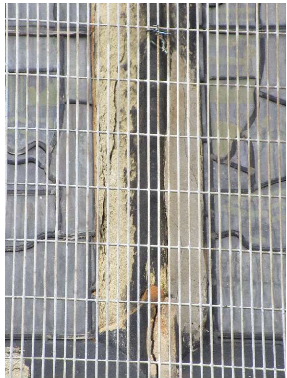
Base of N central mullion
