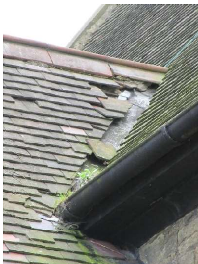
Missing Vestry tiles, plants in silt in the Nave gutter, saplings in corner and ivy getting close to Vestry tiles
