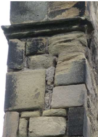
W end – little pointing and stone decay begun
