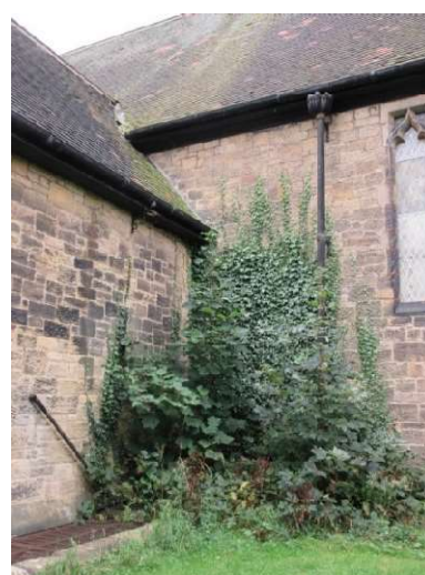
Missing Vestry tiles, plants in silt in the Nave gutter, saplings in corner and ivy getting close to Vestry tiles
