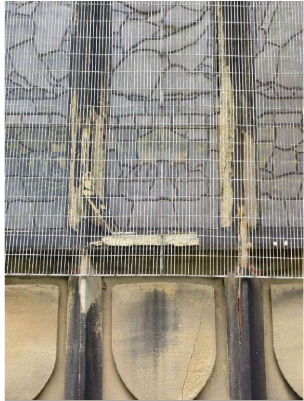
Outside two centre mullions
