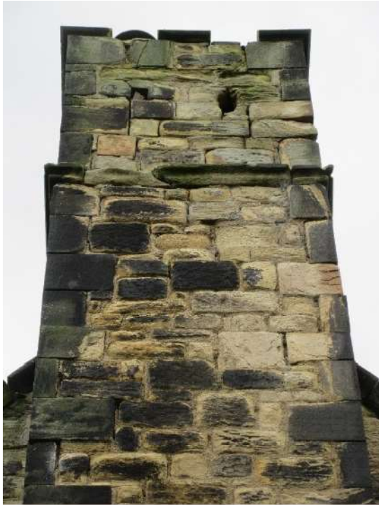
Chimney N side – general decay and daylight through holes both sides of one flue, letting wind through
