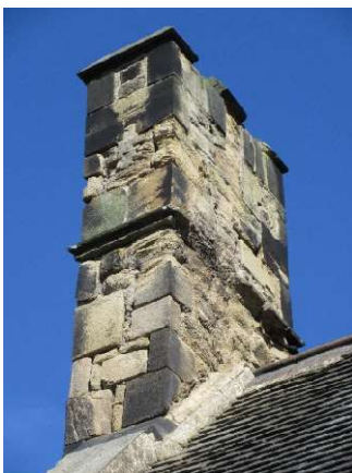
Chimney S and E – widespread decay, part of string course (should throw off water) missing and hole lets wind through
