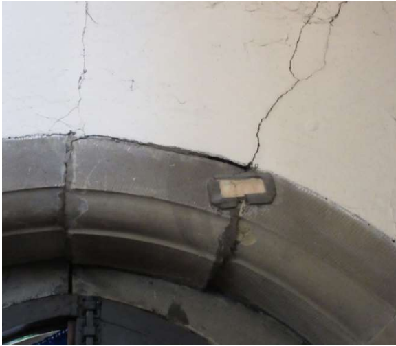
Dropped stone in Porch inner arch
