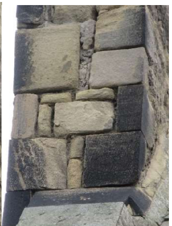
Chimney S and E – widespread decay, part of string course (should throw off water) missing and hole lets wind through
