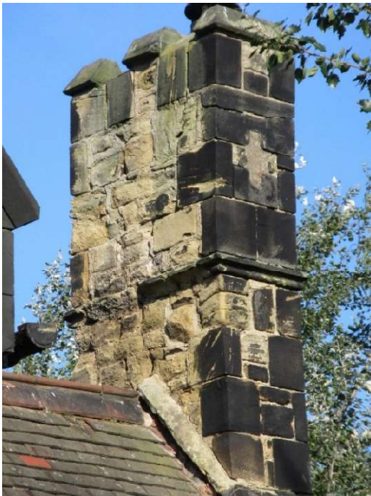
Chimney S and E – widespread decay, part of string course (should throw off water) missing and hole lets wind through
