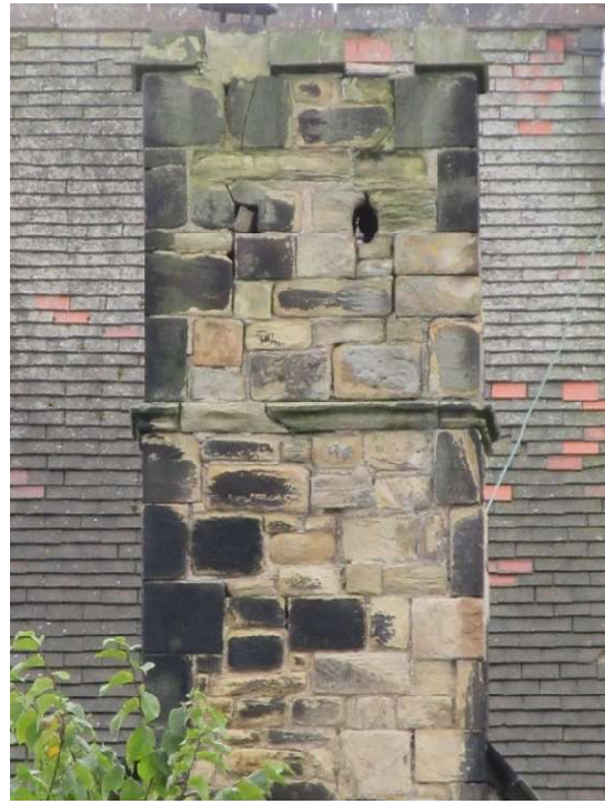
Chimney N side – general decay and daylight through holes both sides of one flue, letting wind through
