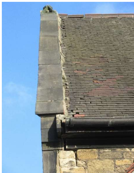
Nave SW gable
