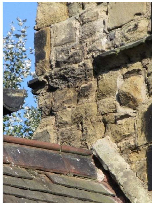
Chimney S and E – widespread decay, part of string course (should throw off water) missing and hole lets wind through
