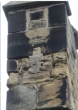
W end – little pointing and stone decay begun
