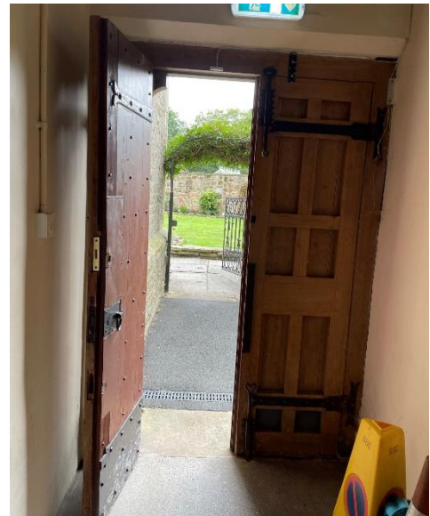
Item 68- South Porch Entrance Doors
