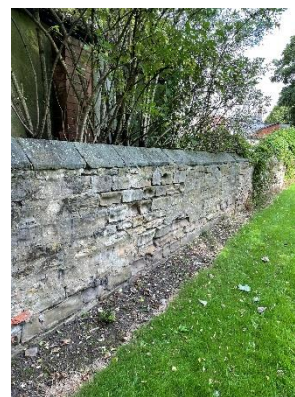
Item 153- Boundary Wall
