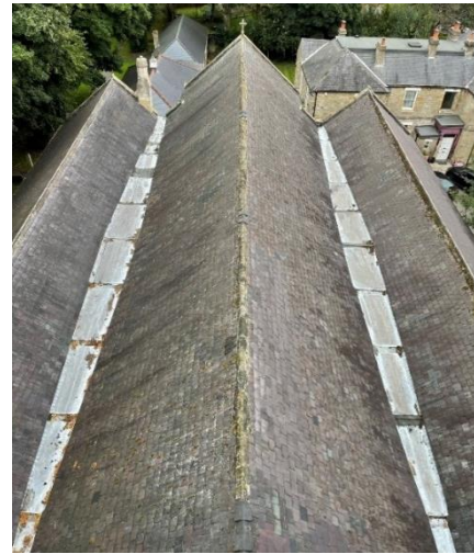
Item 13&14- Roof and Valleys from Tower
