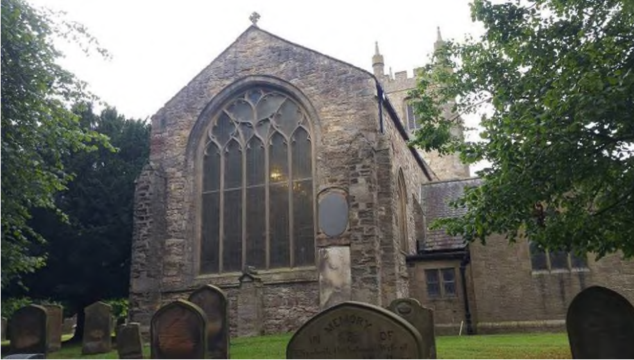
North – Random walling looks ok, relieving brick arch over window is sound.
