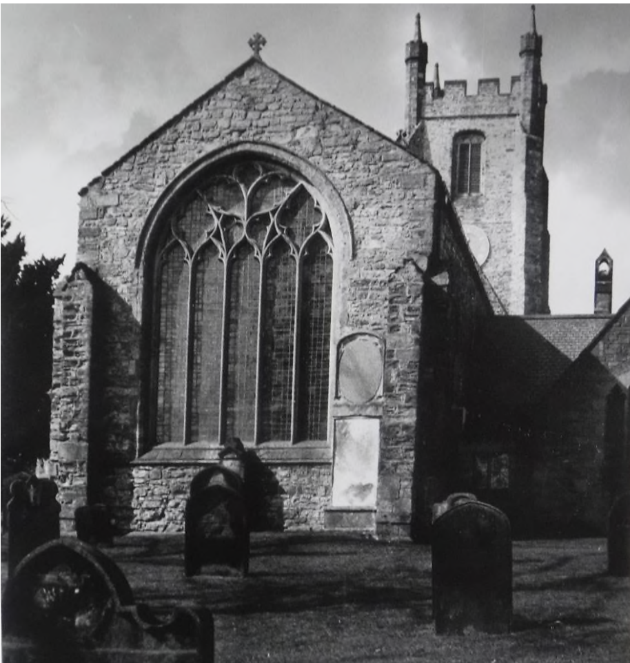
Earlier image, date unknown. Compare erosion on S buttresses
