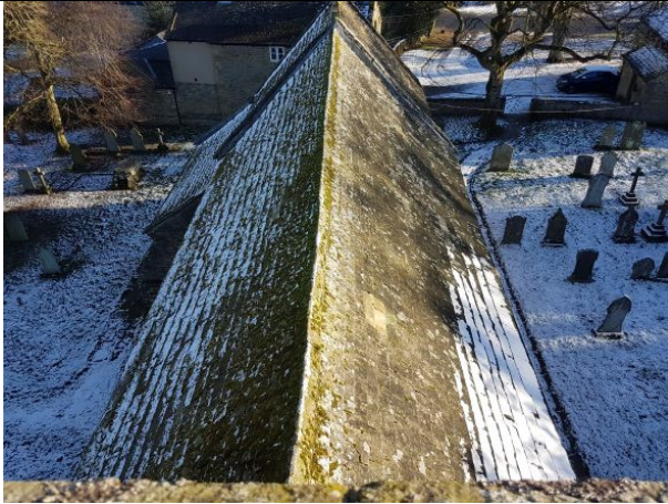
View of Nave and Chancel roofs from Tower
