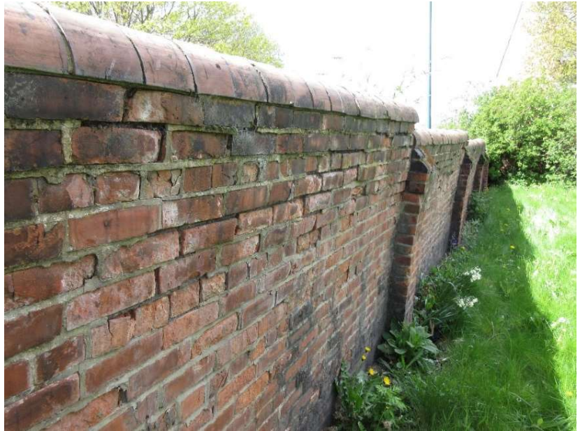
South brick boundary wall decays with significant lean inwards, despite thin piers
