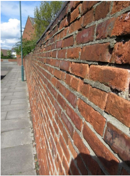
South brick boundary wall decays with significant lean inwards, despite thin piers
