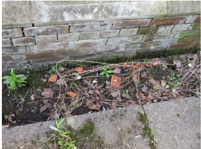
Trench against N Aisle refilling
