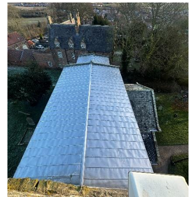
Figure 2- Nave roof from tower
