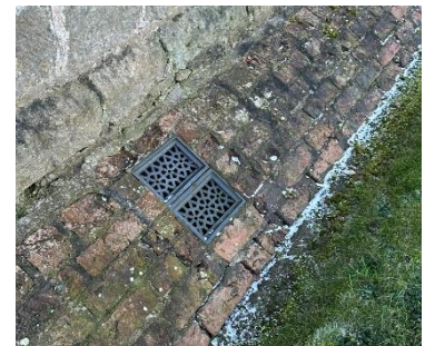
Figure 22- Vents in plinth
