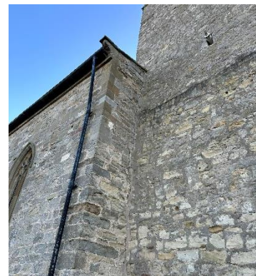
Figure 9 – N joint Tower to Nave
