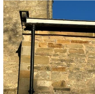
Figure 4 - Gutter to S Nave
