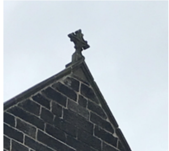
Nave West End Finial Cross
