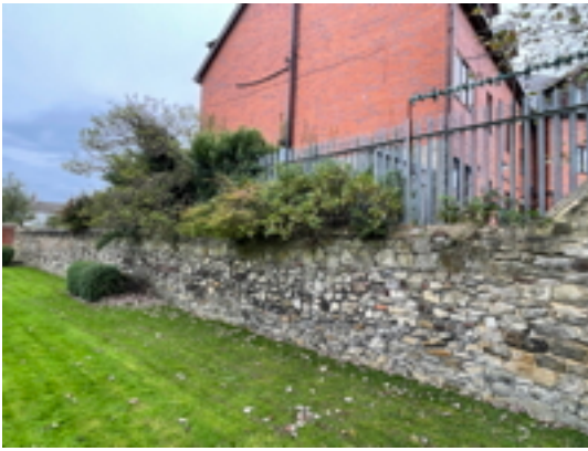
South Boundary Wall East End
