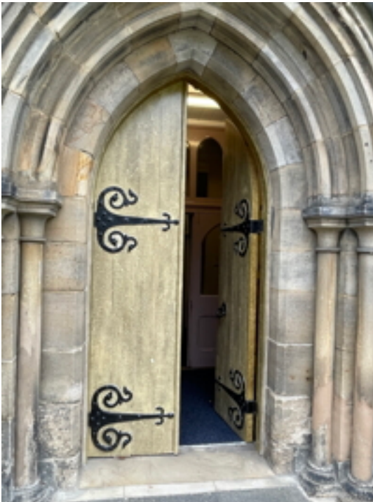
South Porch Doors
