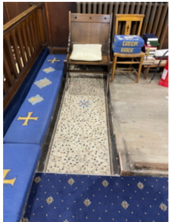
Choir mosaic tiles and timber flooring to pews
