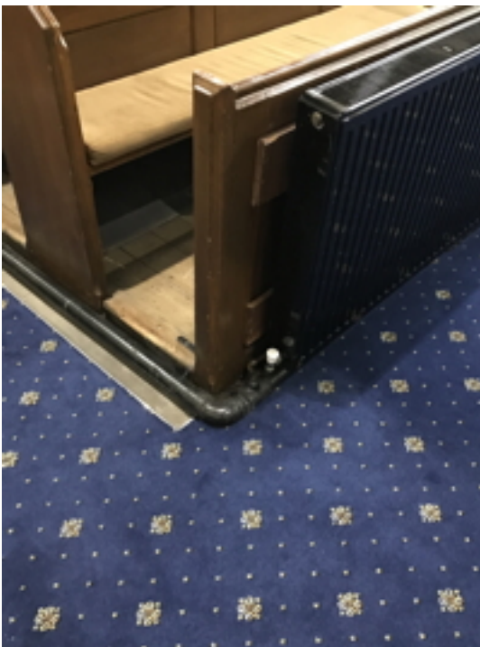
Typical Nave carpeting and timber flooring to pews
