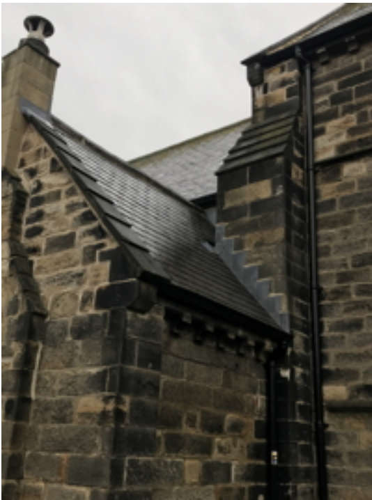
Vestry and Nave Rainwater Pipes and Gutters
