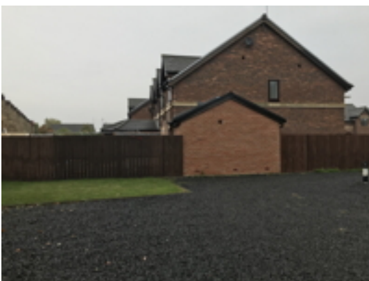
North Boundary Fencing and Garage
