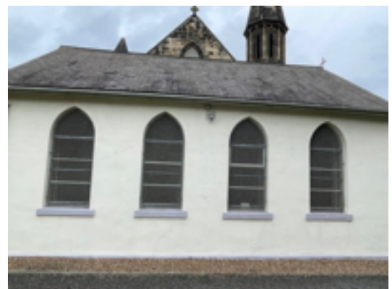
Meeting Room West Elevation Windows
