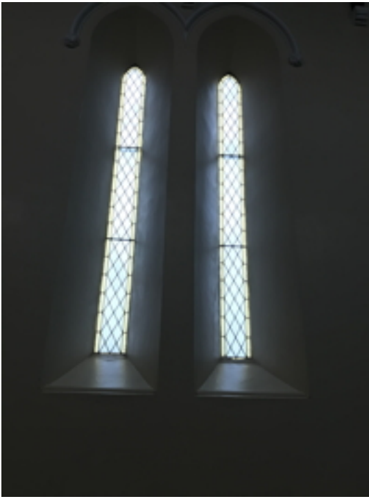
Typical Nave North Elevation Windows
