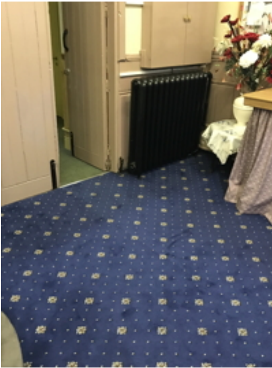
West End Nave Radiator
