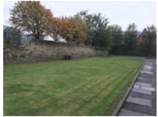
South Boundary Wall West End
