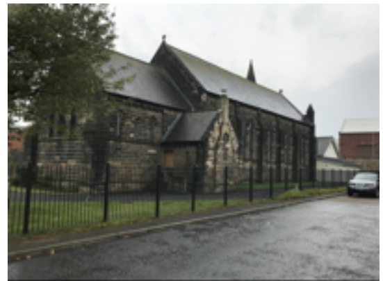
North Boundary Railings
