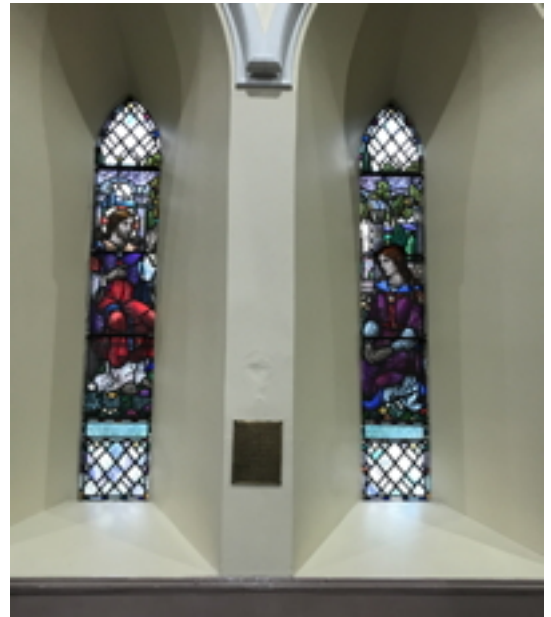
Typical South Aisle South Elevation Windows
