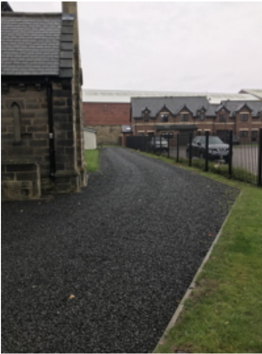
Gravel Driveway to North Elevation
