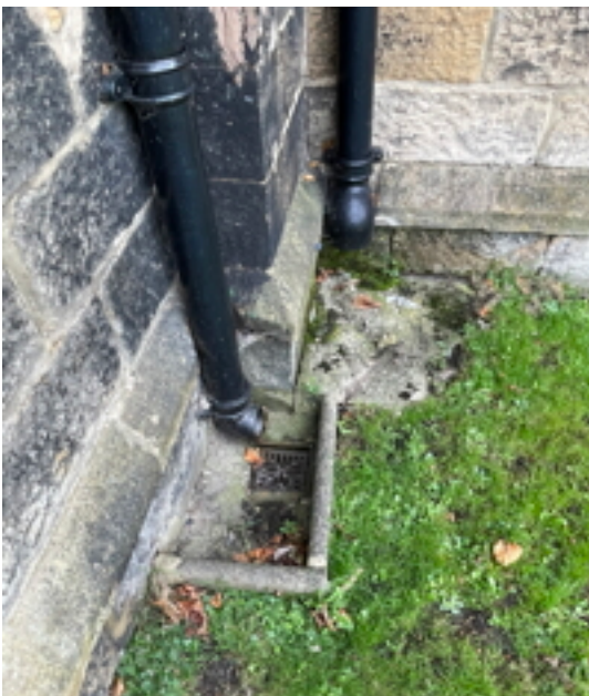
North Elevation Gully
