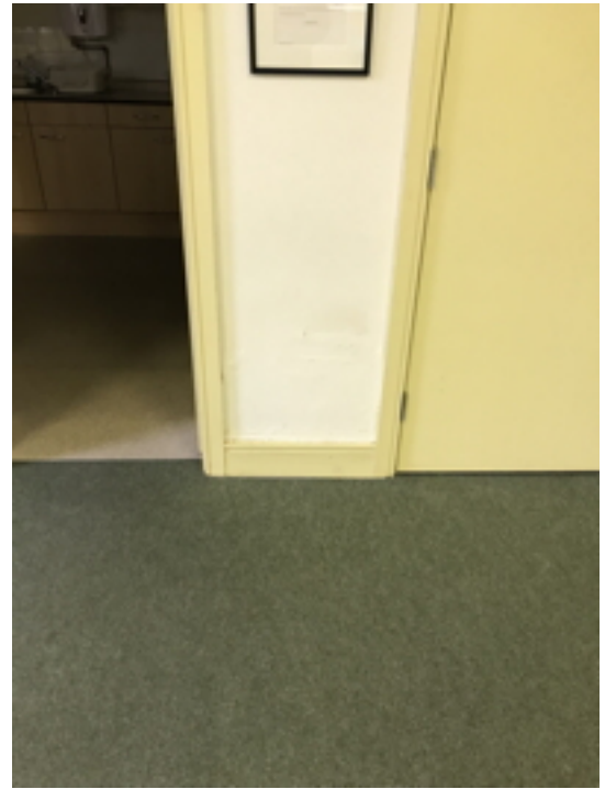
Hall carpeting and sheet vinyl flooring
