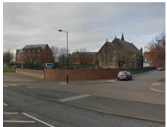
North East Corner Brickwork Wall and Stone and Brickwork East Boundary Wall
