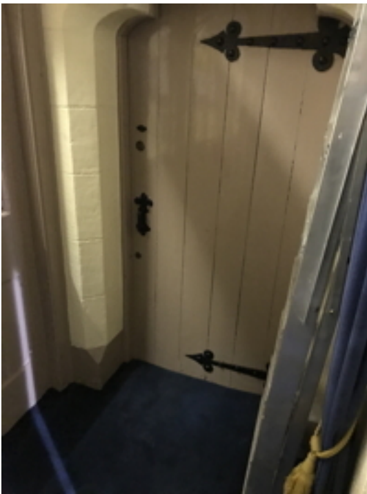
Porch/Tower Staircase Door
