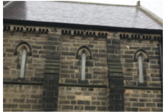
Chancel South Elevation Windows
