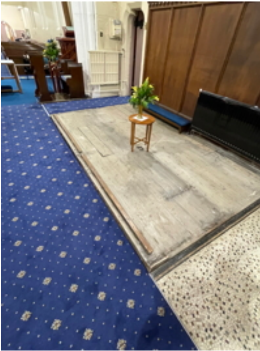
Area where Choir Pews removed with Clergy Seat in Background
