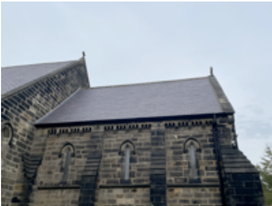
Chancel and Vestry Roofs
