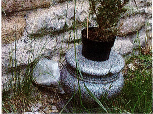
N side – drilled hole loosely plugged by plastic sheeting
