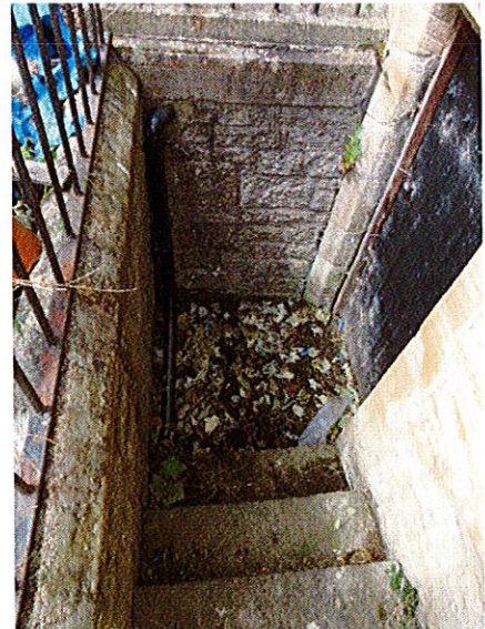
Well at boiler room steps
