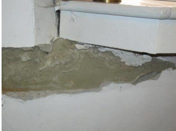
Damaged plaster to North and East walls in Vestry
