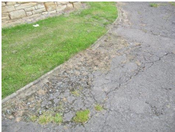
Grass growth and cracked tarmac to West and south side of the church on the main access route
