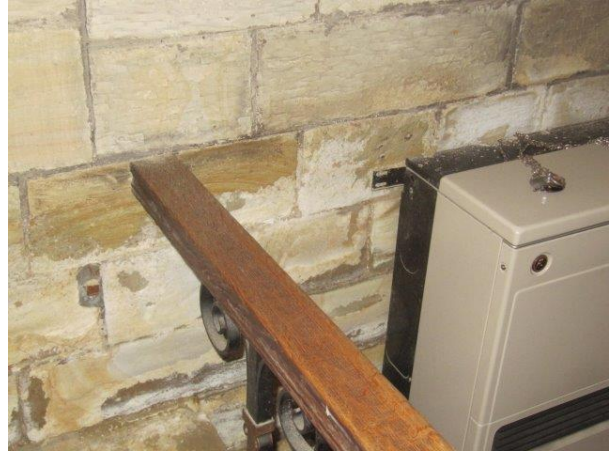
Damaged stonework and salt efflorescent to North wall of Chancel
