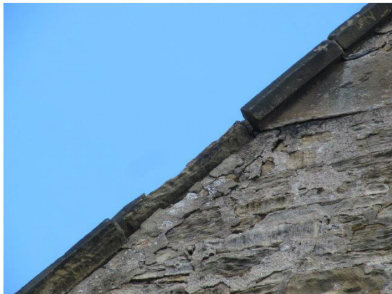
Damaged section of water table, cracking mortar, open joints and weathered stonework to West Elevation of Nave
