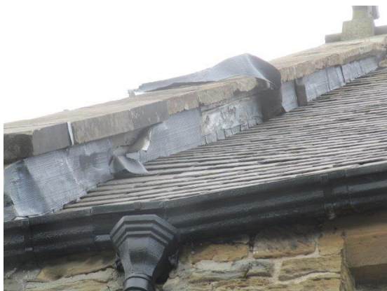
Lifted and damaged flashings to North Nave roof Slipped slates to South Aisle roof
