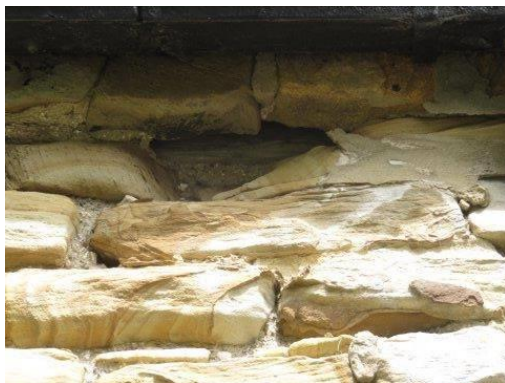
Weathered stonework exposing wall plate and loose/missing stonework to East end of South Aisle
