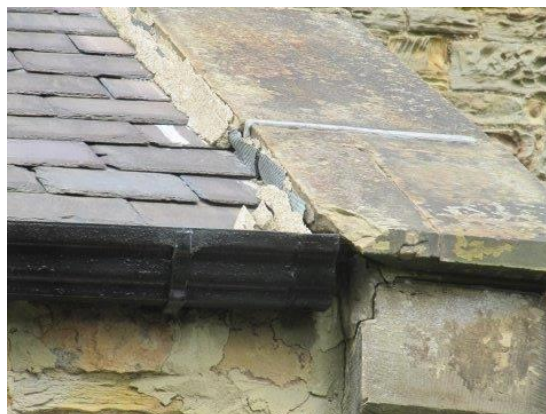
Missing and cracked mortar fillets to roofs on South Elevation
