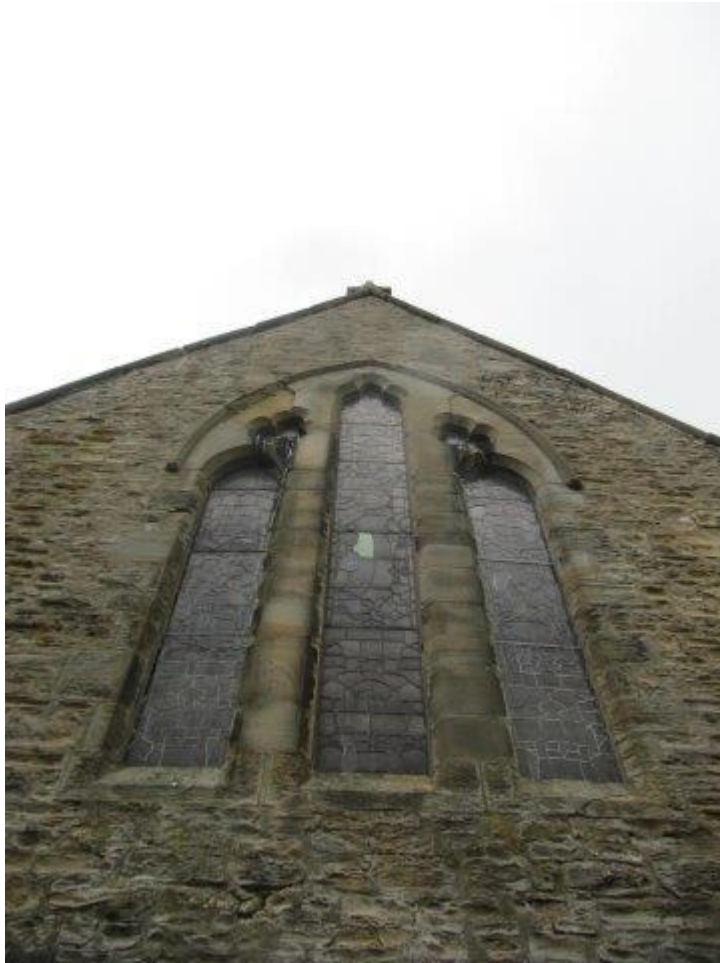
East Elevation of Chancel
