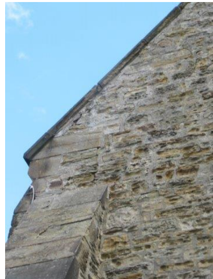
Damaged section of water table, cracking mortar, open joints and weathered stonework to West Elevation of Nave
