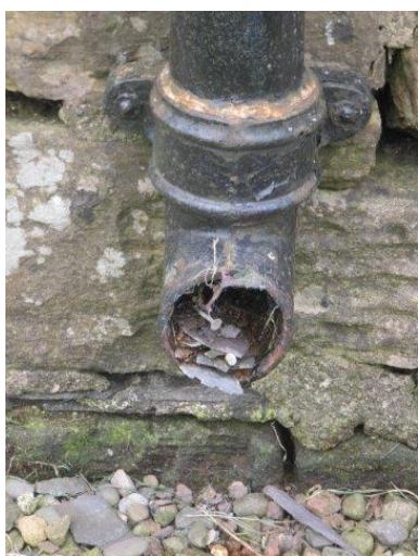
Slate fragments in shoe to downpipe on North Elevation of North Aisle
