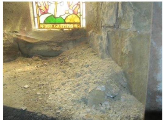
Sanding stonework to South Organ Chamber
