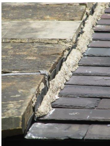
Missing and cracked mortar fillets to roofs on South Elevation
