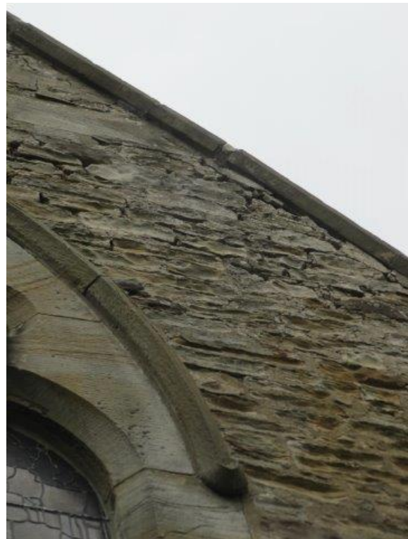
Open joints, cracking and damage to stonework to the east window, East elevation of
