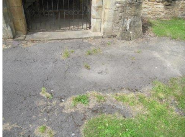
Grass growth and cracked tarmac to West and south side of the church on the main access route
