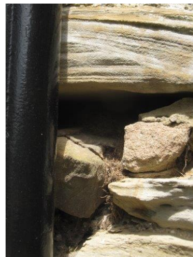
Weathered stonework exposing wall plate and loose/missing stonework to East end of South Aisle
