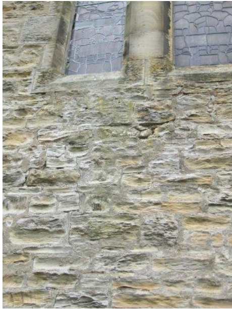
Cracking and missing mortar to East Elevation of Chancel under the window
