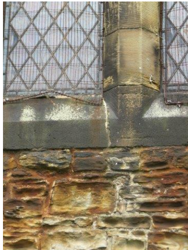
Open joint to water table and cracked mortar under to East Elevation of South Organ Chamber
