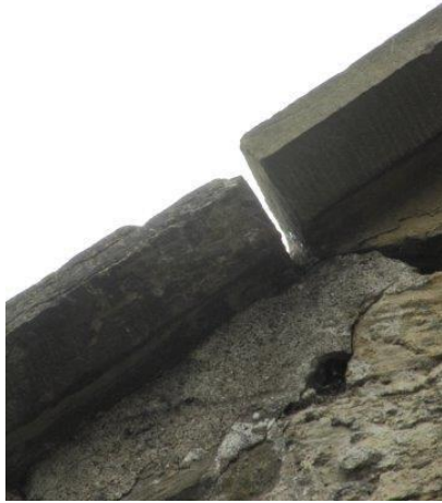
Open joint to water table and cracked mortar under to East Elevation of South Organ Chamber
