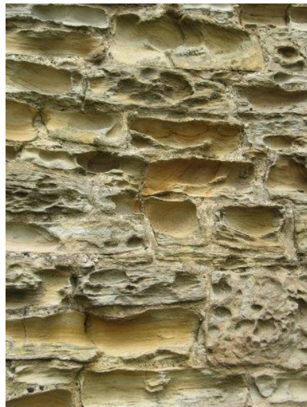
Open joints and cavities to West Elevation of South Aisle
