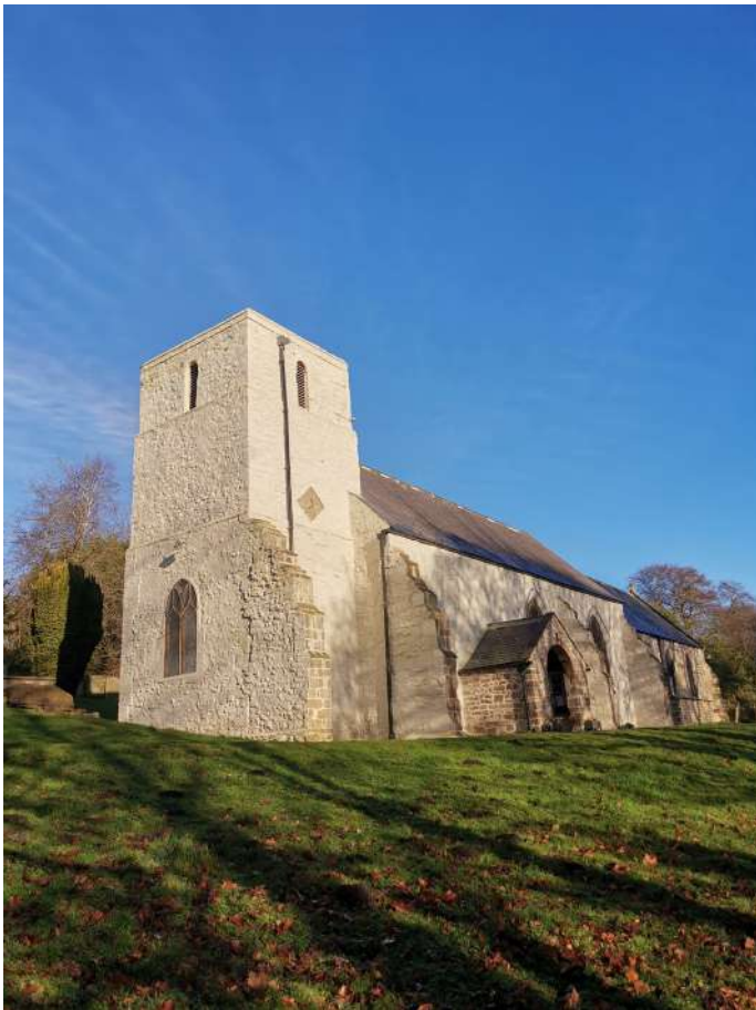
Stone consolidation to tower and buttresses
