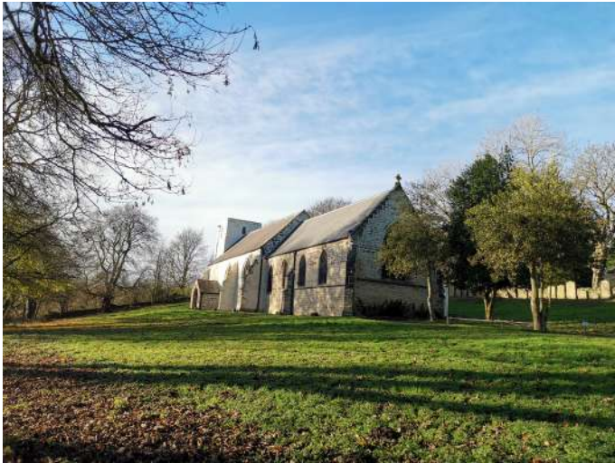
Churchyard cleared of headstones. Some stacked up along northern boundary wall
