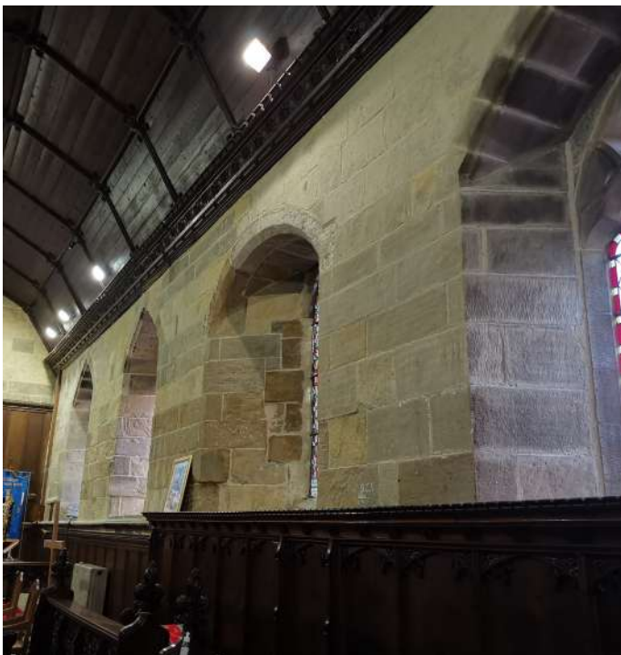
Internal chancel masonry has been cleaned, repaired and re-pointed
