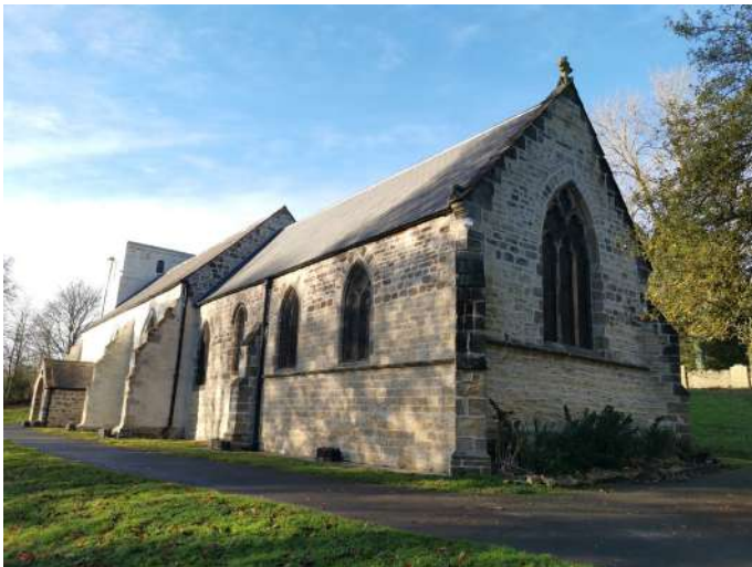
South eastern of chancel - new roof and apex cross
