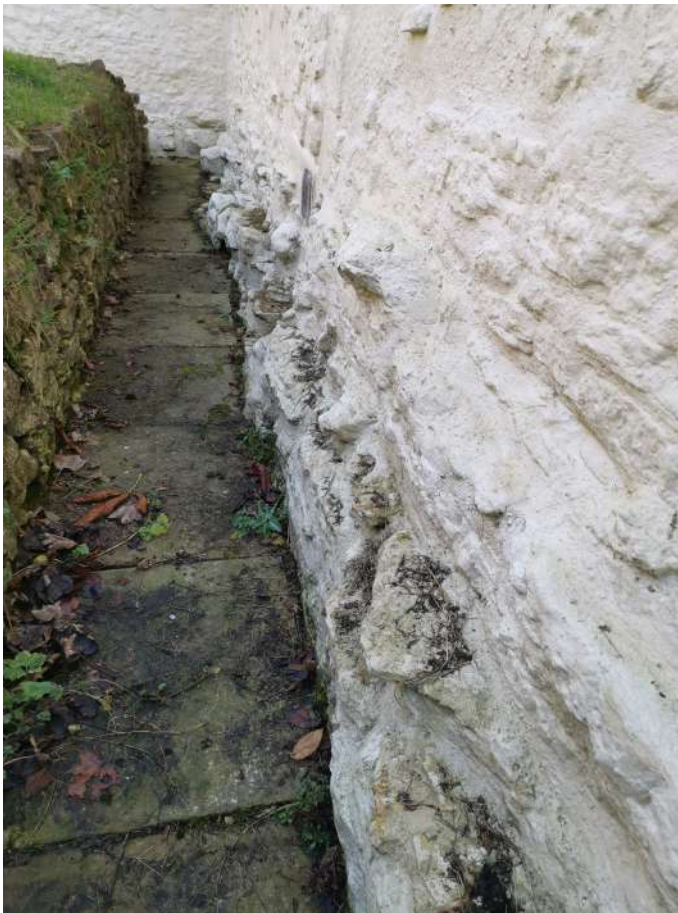
Exposed foundation stones to north of tower
