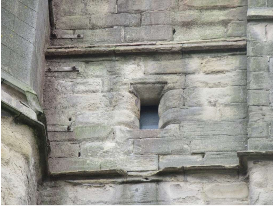
Masonry at E windows
