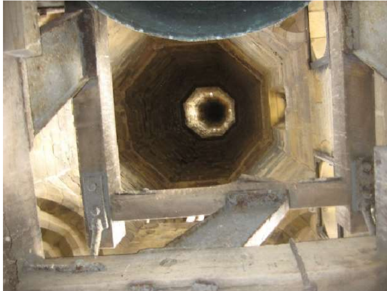
Upwards from Belfry through bell frame into spire
