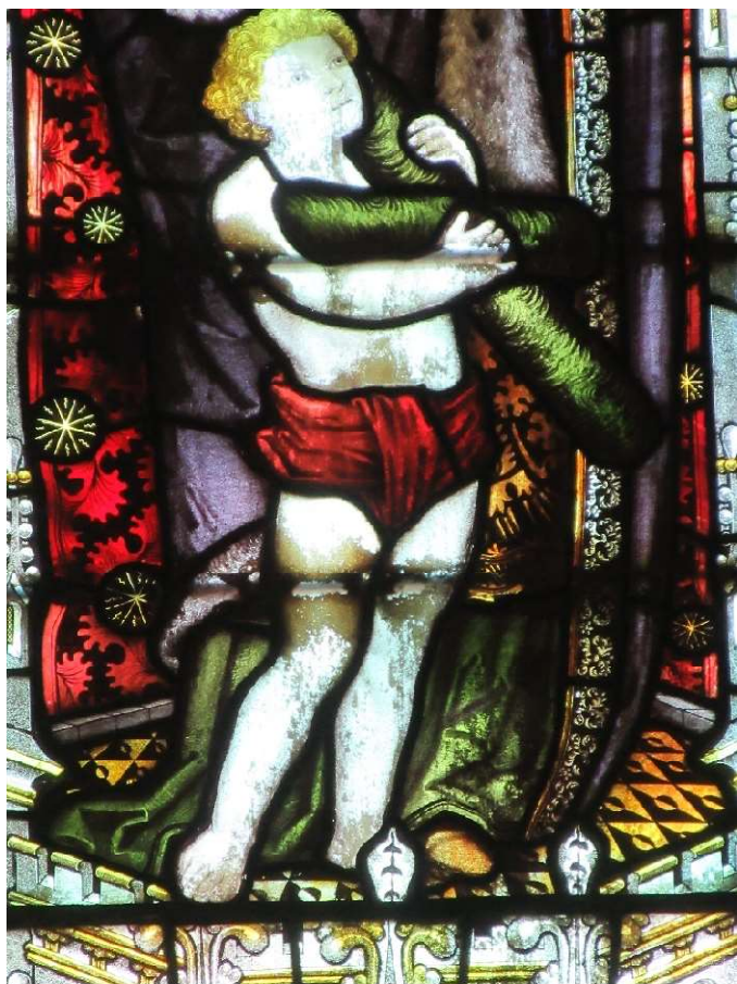
N Chancel – some loss of paint at figure
