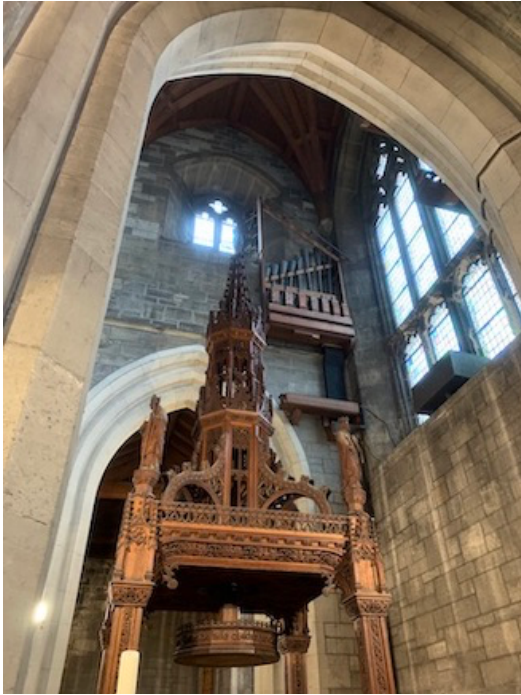
33. Tower Base – looking south towards entrance
