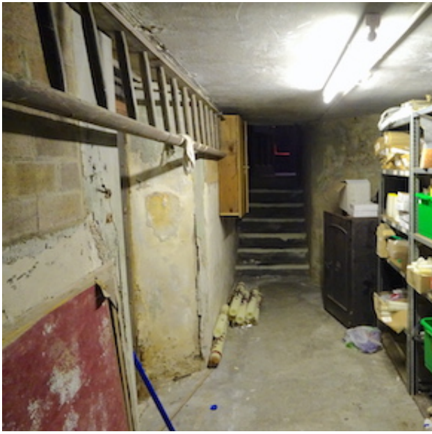
45. Passage (old Vestry entrance on left) below Chancel
