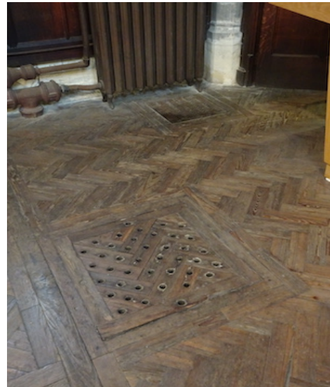
44. North Aisle – vented timber cover to heating pipes below
