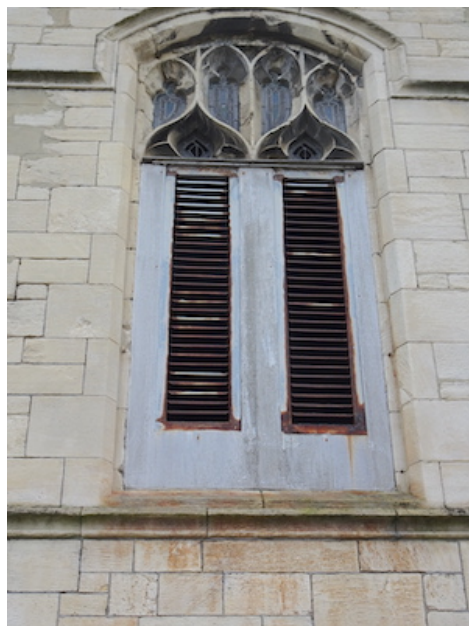
14. North Porch north face – blocked window opening.
