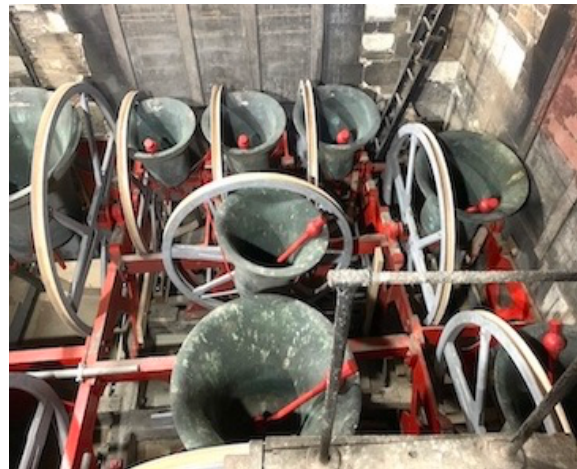
31. Tower Belfry – bell frame and bells
