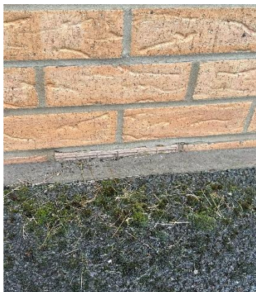
Figure 5 – Air Brick to South
