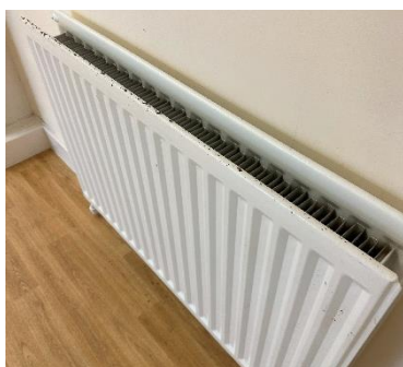
Figure 14 – Radiator Rust
