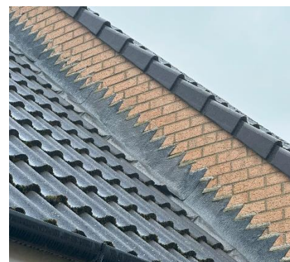
Figure 2 – East Abutment Flashing Lifting
