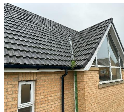
Figure 1 – West Hall Valley
