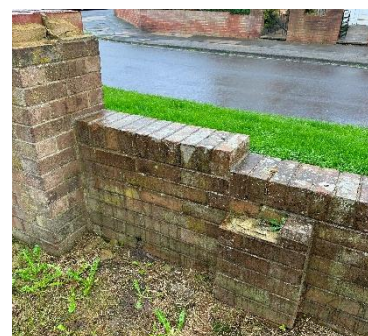
Figure 17 – Boundary Wall Pier
