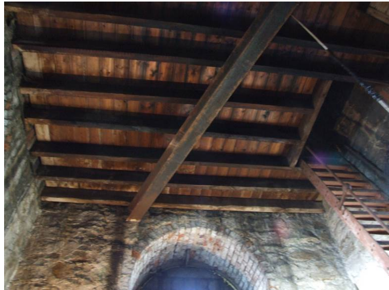
Transverse steel beam in 'clock' chambers
