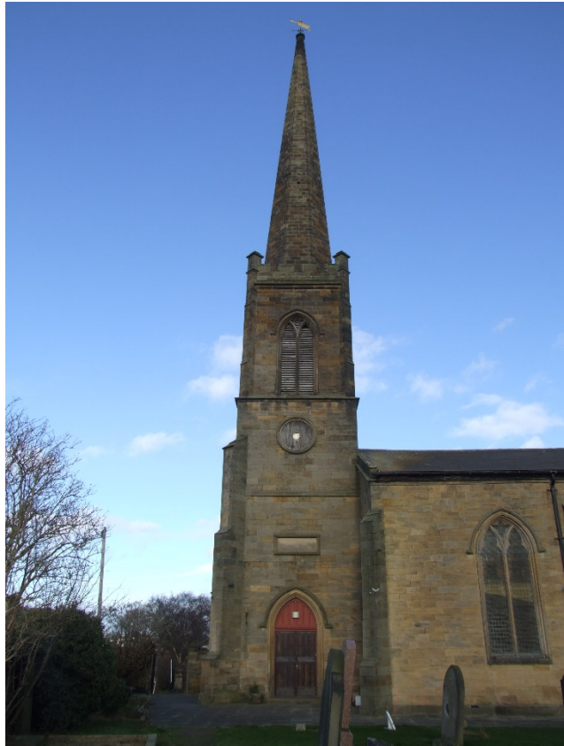
Tower; south elevation
