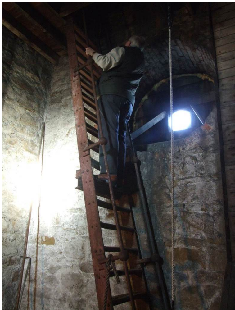
Steel ladder to bell chamber
