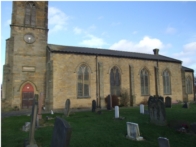
Nave; south elevation
