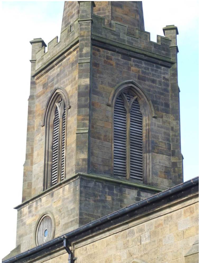
External view of tower levels
