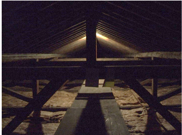
Insulated ceiling above nave
