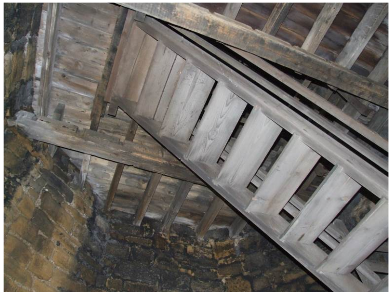
Underside of parapet floor
