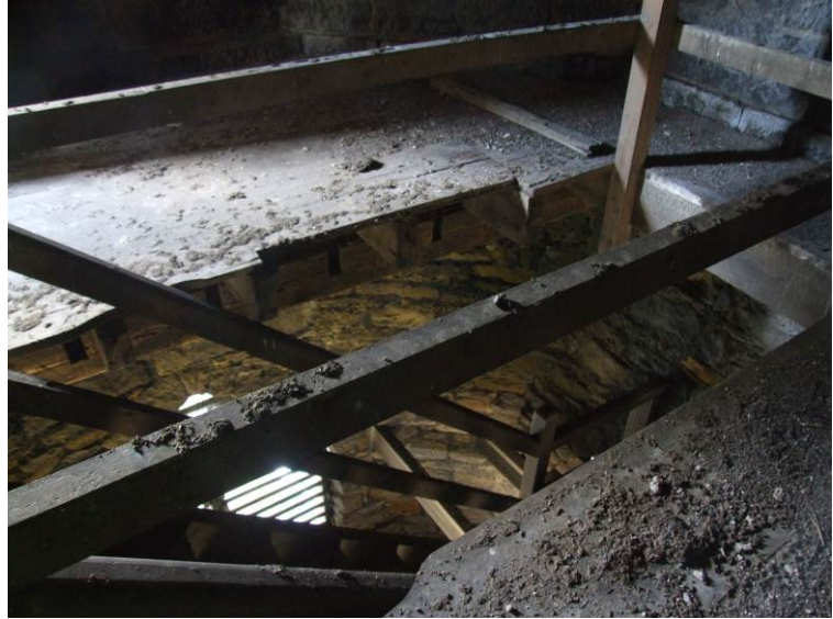
Parapet level floor with stairs down
