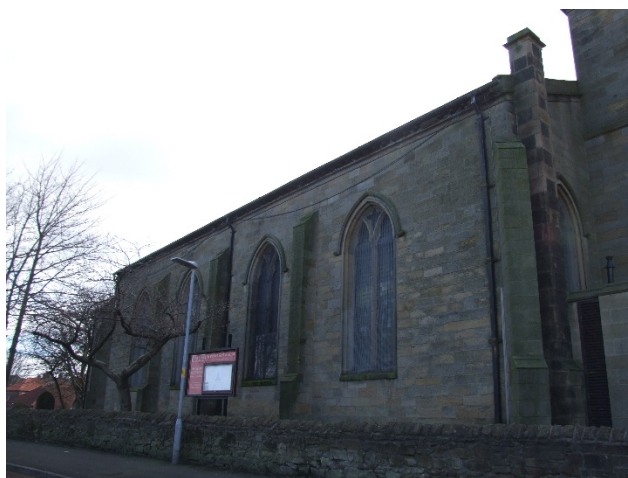
Nave; north elevation
