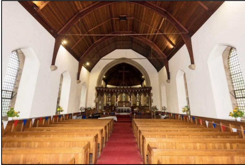
Nave looking east
