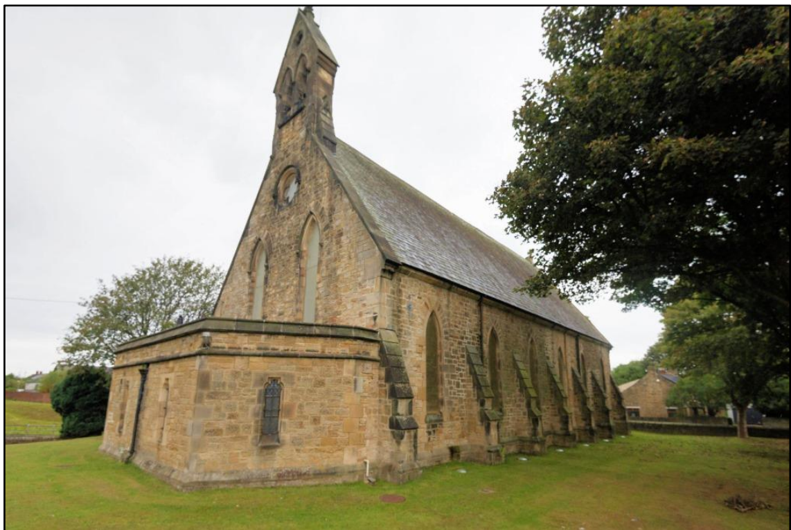
West Elevation from the southwest
