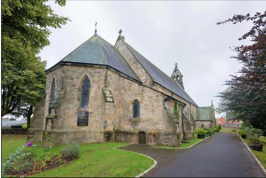
View from the northeast
