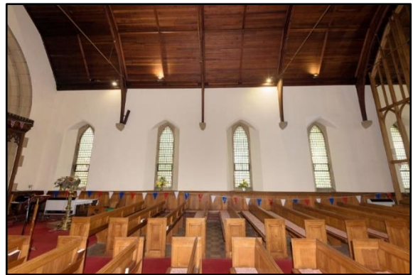
Nave looking north
