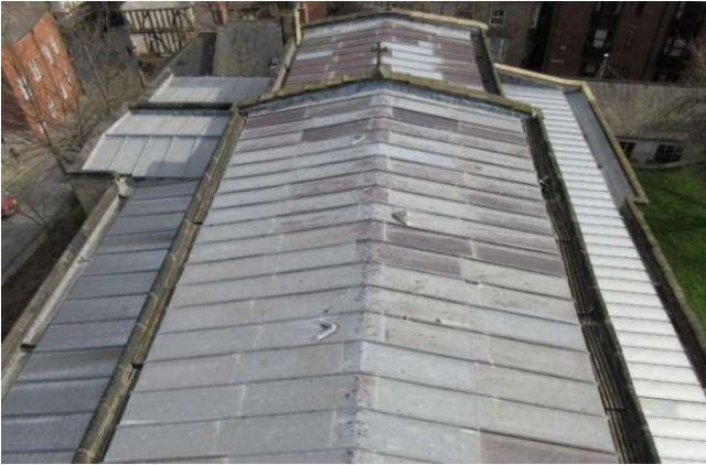
Roofs from W Tower
