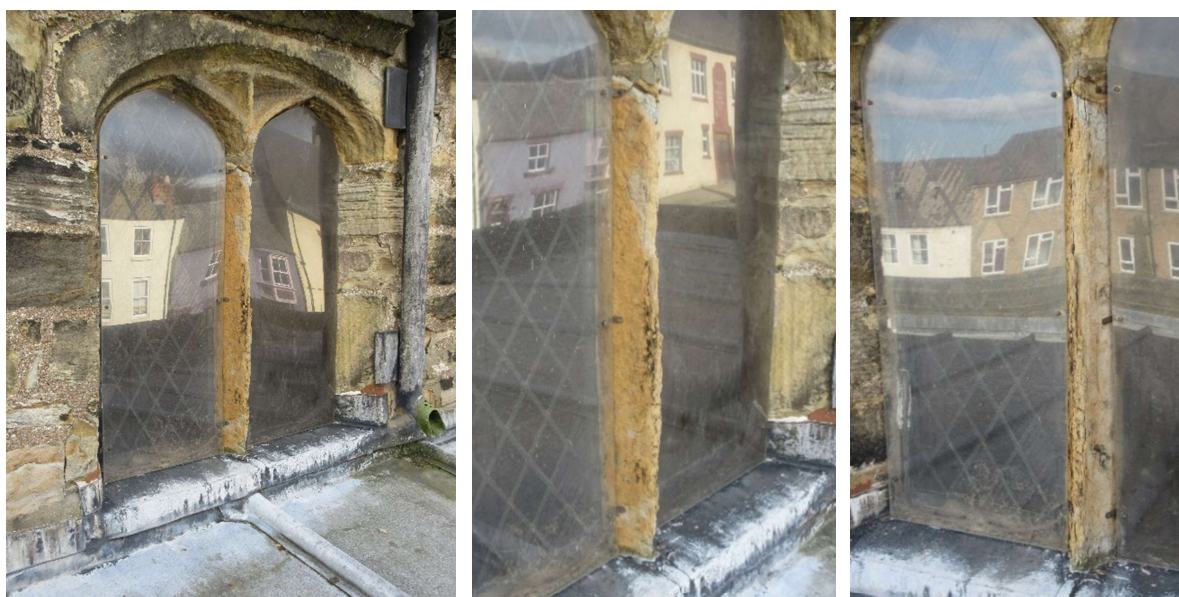
Nave NW clerestory
