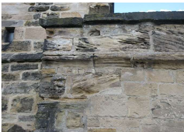
W end of Nave S clerestory parapet
