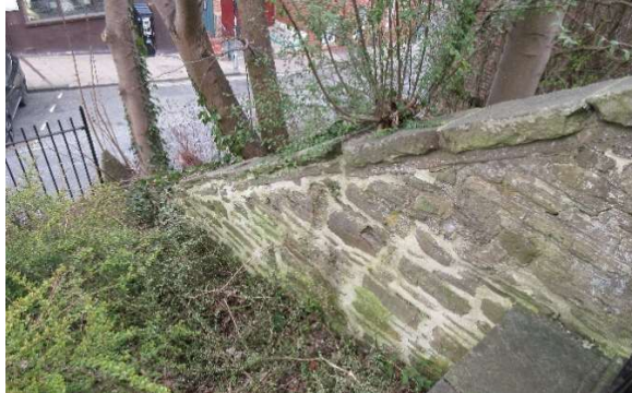
N end of E retaining wall
