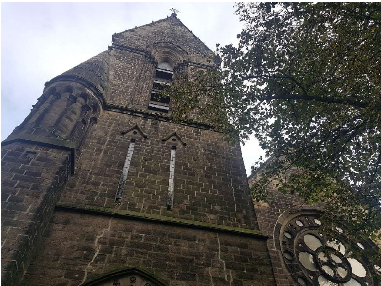
Fig. 4 | Church Photographs (4.1 + 4.2 Exterior)
