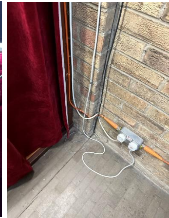
Figure 34 - Hanging JB as 16.2 Figure 35 - loose wire
