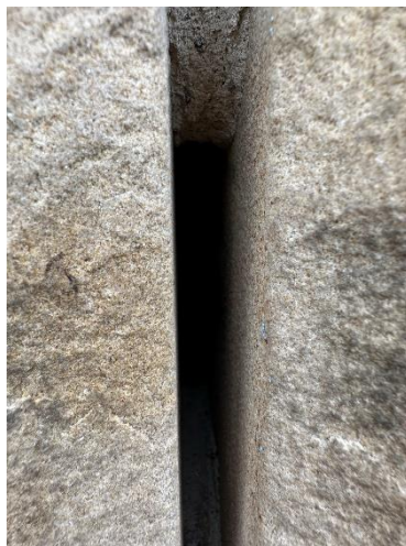
Figure 19 - open joint to cavity
