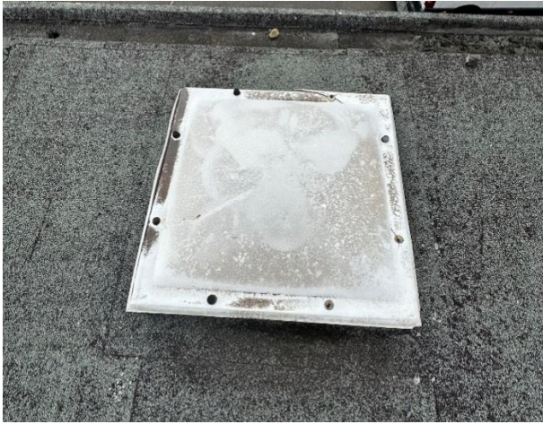
Figure 6 - Rooflight 19 - cracked
