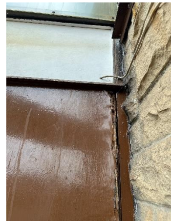
Figure 28 - Weathered frame
