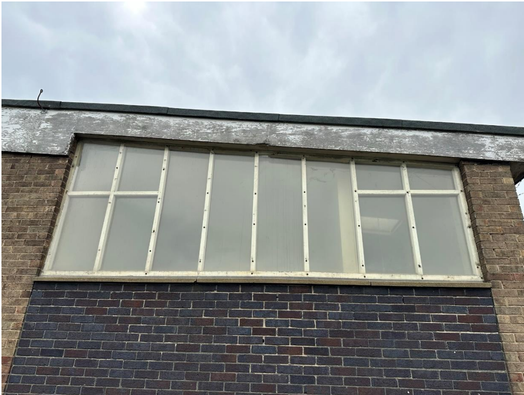
Figure 29 - Large high-level windows to NW
