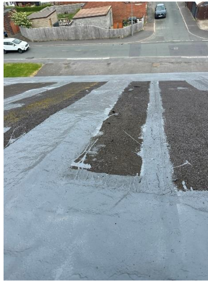
Figure 12 - Central E view
