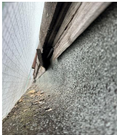
Figure 9 - Underside of slipped glass
