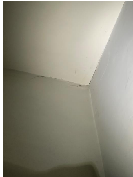
Figure 31 – Boiler room ceiling as item 9.6
