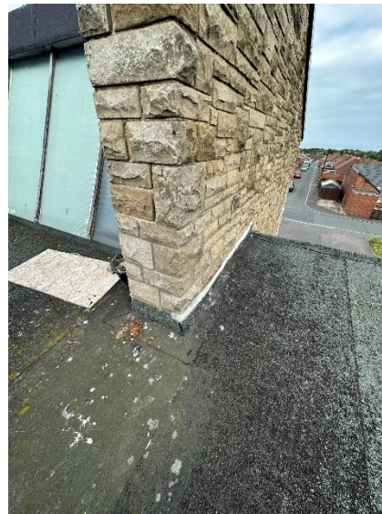
Figure 5- S. felt upstand.
