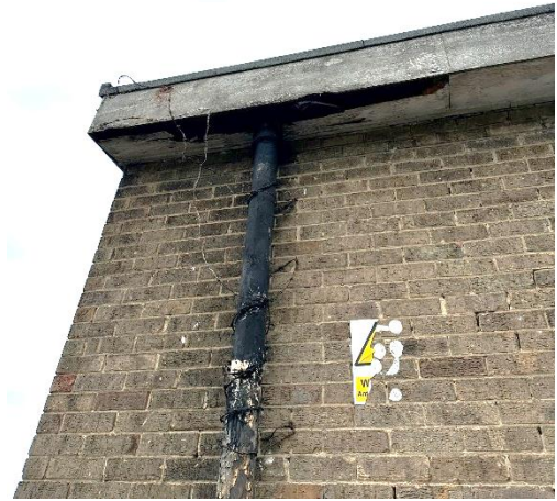
Figure 7 - NW soffit as item 2.5
