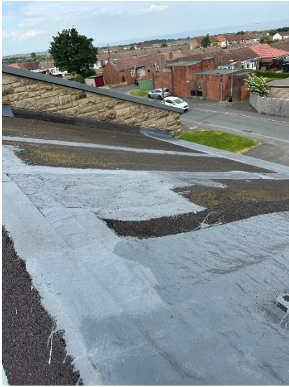
Figure 11 – N side of sanctuary roof
