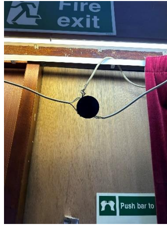
Figure 34 - Hanging JB as 16.2 Figure 35 - loose wire
