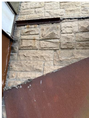
Figure 27 - Mastic to wall
