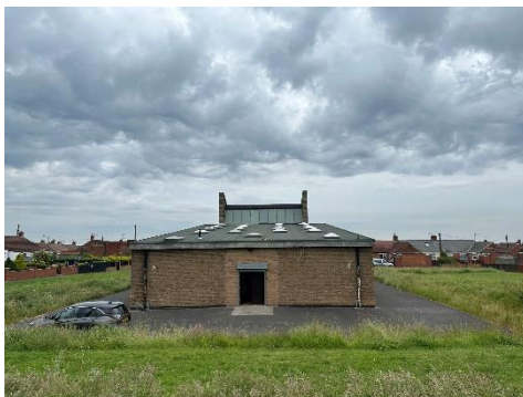
Figure 1 - External entrance view
