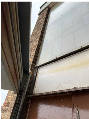
Figure 26 - Former canopy seating
