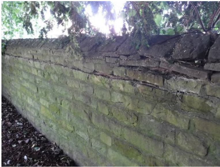
Root encroaching into the wall head breaking the stones
