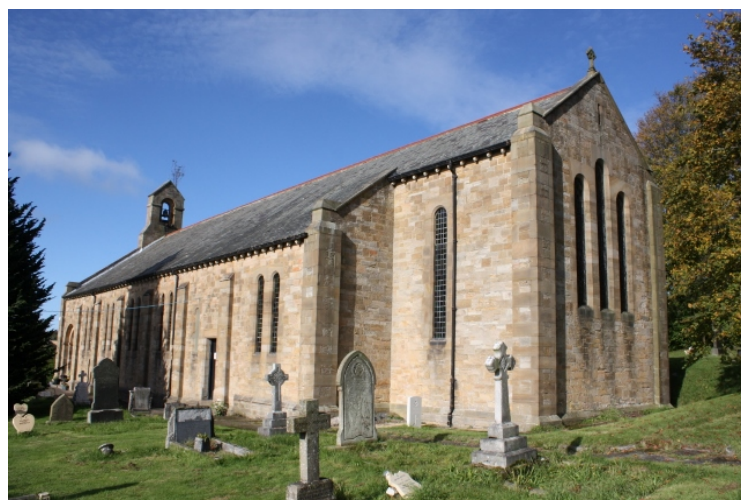
View of church from South East
