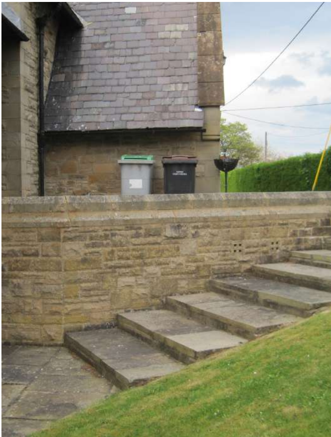
Vent to the former boiler room in wall adjacent to the steps - keep clear
