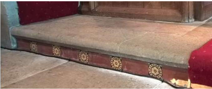
Encaustic tiles in riser of chancel step in good condition
