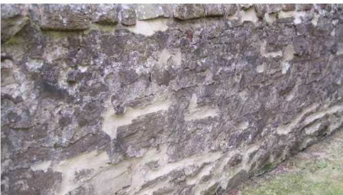
Boundary walls recently patch pointed with cement mortar.
