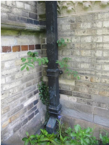
Ivy and saplings to West Elevation of the Porch
