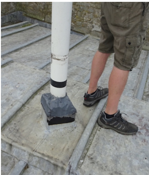
Tower roof – plastic 'sleeve' on flagpole base
