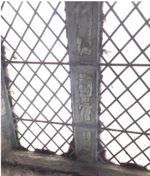
Tower intermediate chamber – west window mullion
