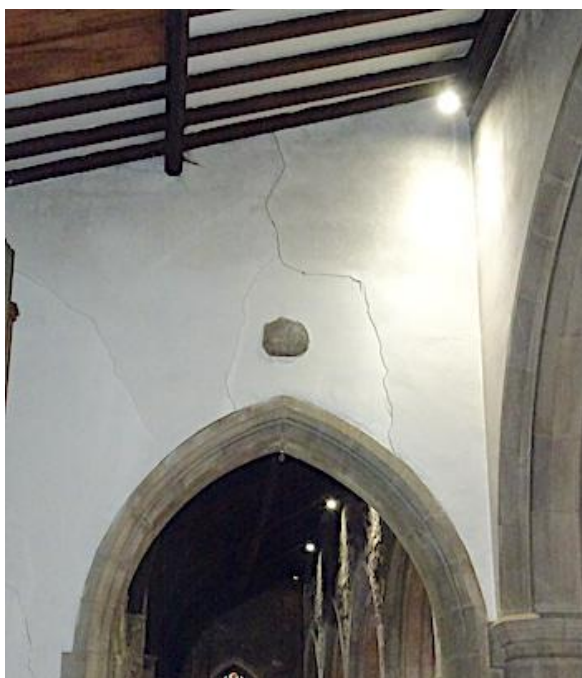
28. and 29. North Chancel Aisle – fractures in South Transept wall above and to side of arch.
