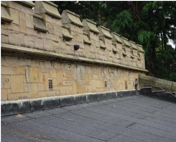
5. South Chancel Aisle roof and Chancel South wall stonework
