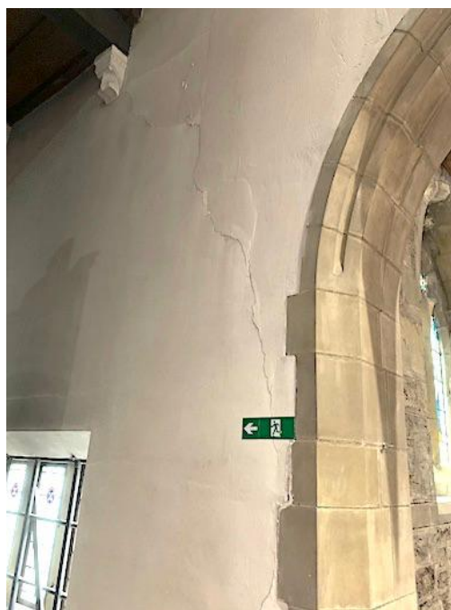
28. and 29. North Chancel Aisle – fractures in South Transept wall above and to side of arch.
