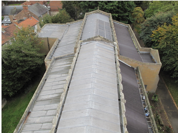
01 General view of roofs looking east from Tower
