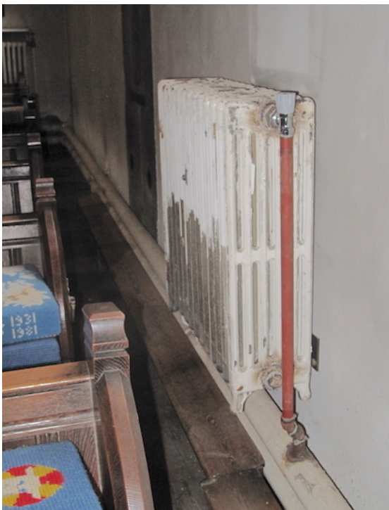
34 North Chancel Aisle – undecorated radiator and pipes
