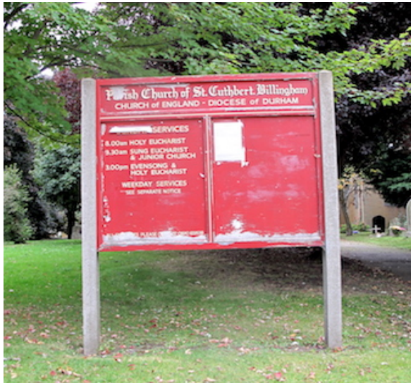
24 Notice board – some repainting needed
