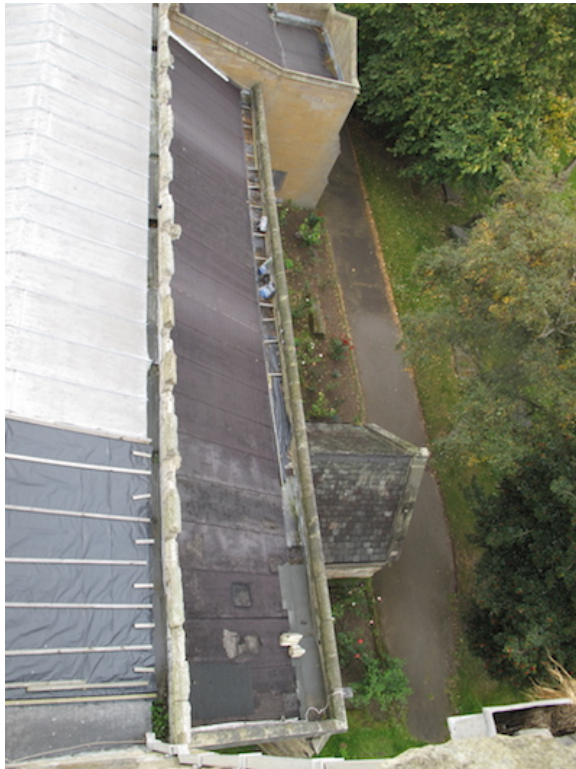
07 Nave Roof and South Nave Aisle Roof
