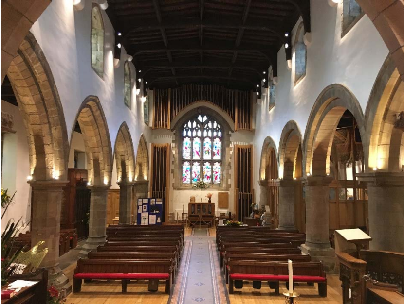
Photo 26 Internal view looking west.
