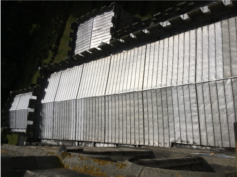
Photo 3 Nave, Chancel and South Transept roofs from Tower.
