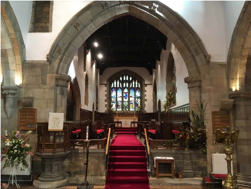
Photo 27 Internal view looking east.
