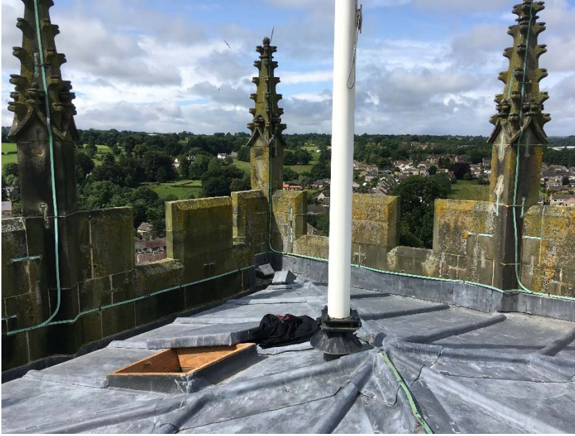
Photo 2 Tower roof, pinnacles, lightning conductor, hatch and flag pole from northeast.
