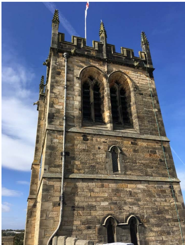
Photo 11 Upper Tower east elevation with lead RWP and lightning conductor.
